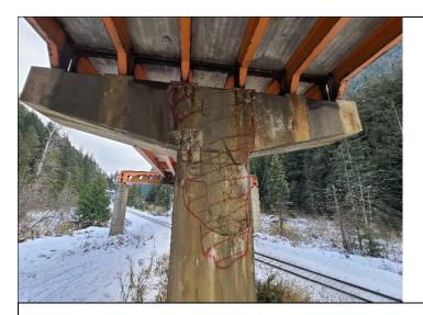
Partial Depth Patch Bent Repair (Bent 5 shown)
