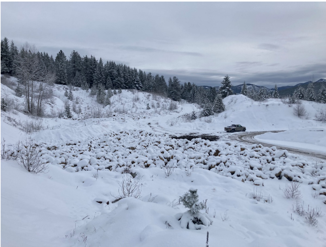
View looking east at riprap and ditching that needs to be moved to mine the suitable material underneath. December 2021.
