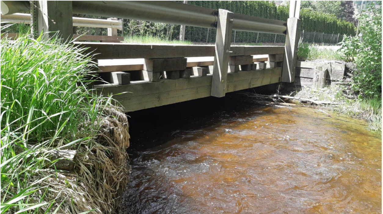
Photo 1 Creighton Road Bridge (Structure No. 06486)
