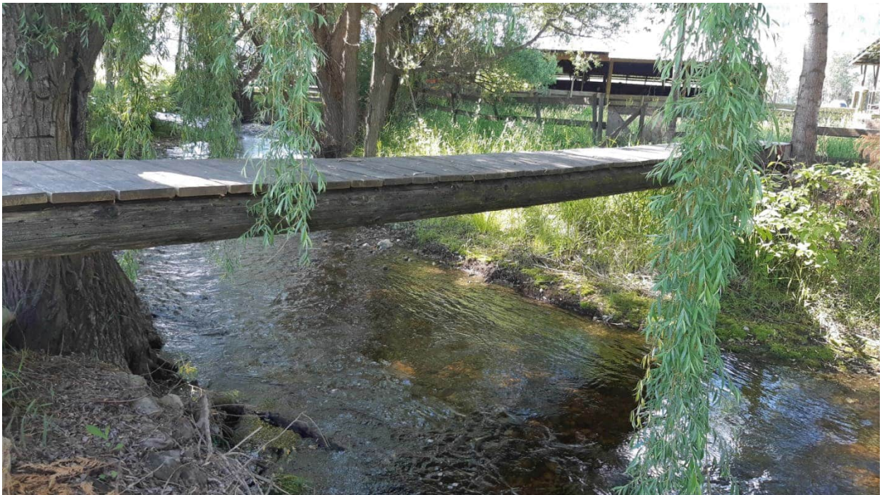
Photo 2 Pedestrian Bridge No. 1 (Upstream of Creighton Road Bridge (Structure No. 06486))
