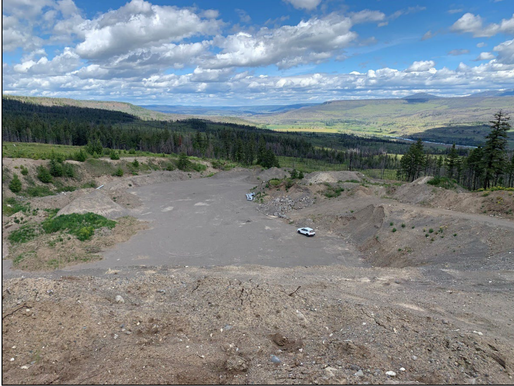
Figure 1 View from the top of the face looking down at the pit floor where there is room for crusher setup and stockpiling (July 2022).
