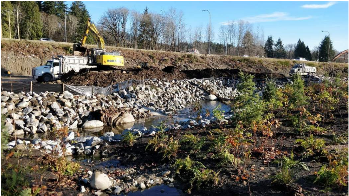
Figure 4-4c: Riffle-pool 3 months post construction with LWD, root wads and habitat boulders.
