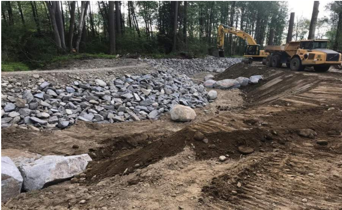
Figure 4-4a: Shaped pool during construction. Habitat boulders and weir crest rocks visible.
