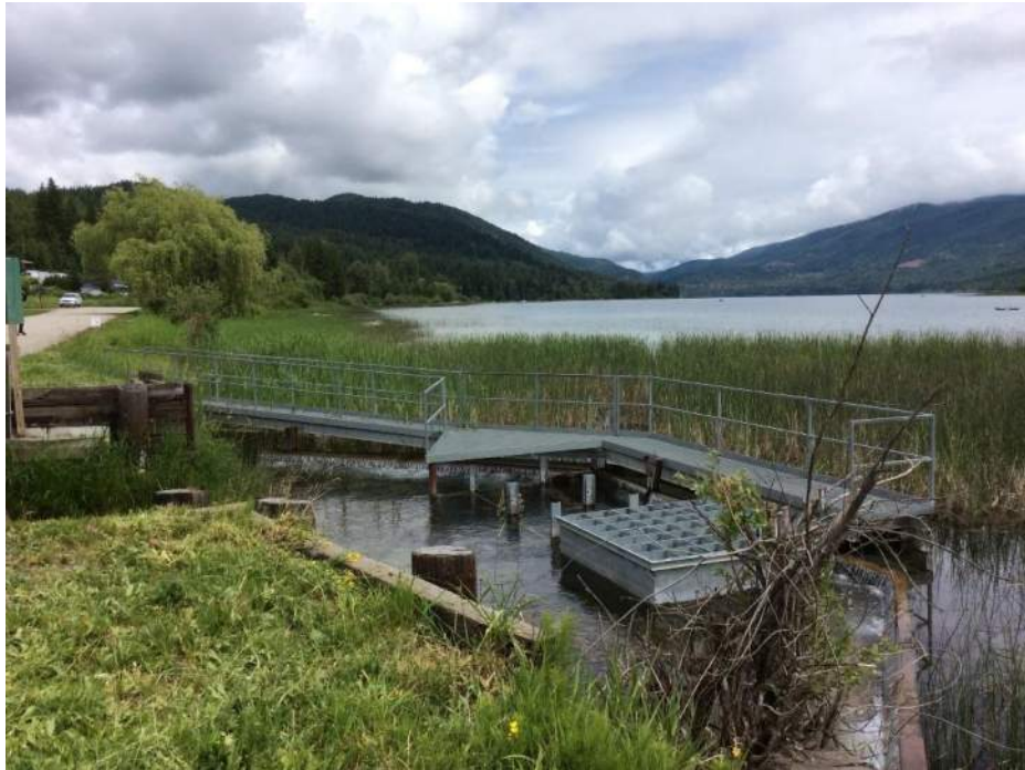
Figure 3-3: White Lake Outlet Control Structure
