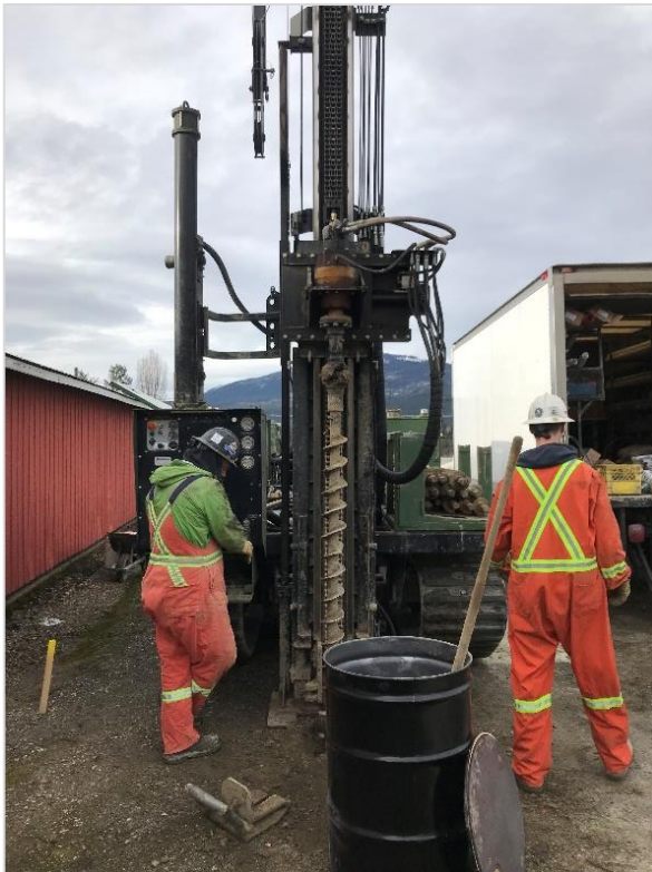
Photograph 3 –Drilling MW18-A1-02 using the track mounted auger rig. Looking north.
