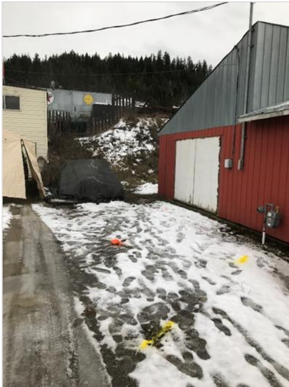
Photograph 1 – Typical 5 x 5 m utility clearance area at selected drilling locations (orange paint denotes the limits). MW18-A1-01 location, looking southeast.
