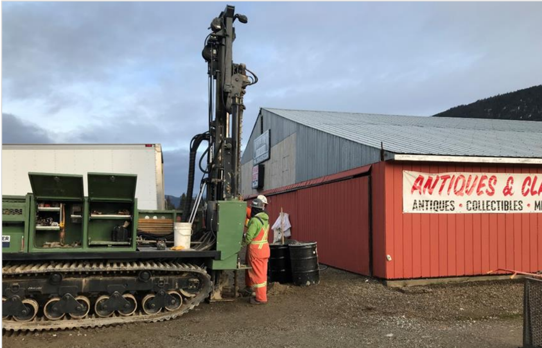
Photograph 3 –Drilling MW18-A1-02 using the track mounted auger rig. Looking north.
