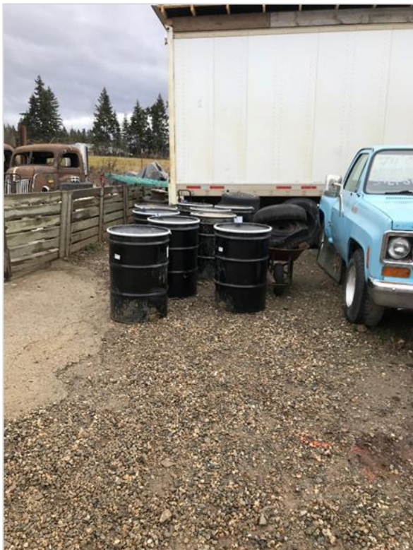
Photograph 6 – Drill cuttings were placed in sealed labelled drums on Site for future disposal. Looking south.
