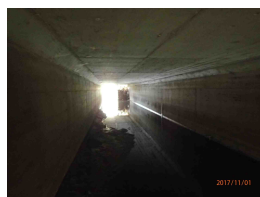
Filename: 2017 roof and sidewalls.JPG
