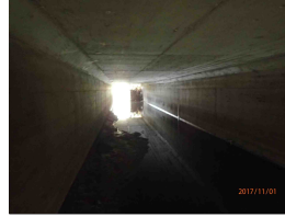
Filename: 2017 roof and sidewalls.JPG
