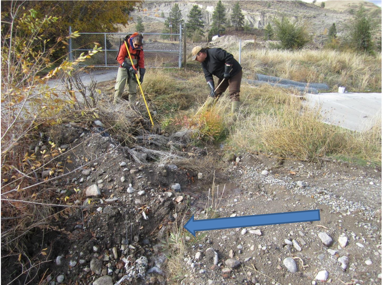
Photo 4-2: Construction alteration of Skaha Creek above Highway 97 at Site 2. Slumping, erosion, and sediment transport has occurred, indicated by the blue arrow.
