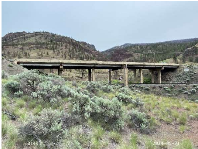
01491 2024-05-21 North Looking South
