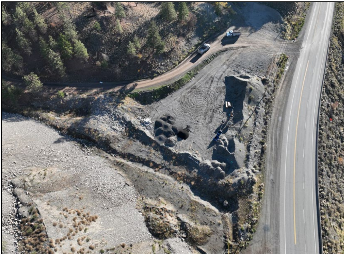
View of lower bench/crusher setup area, and access (November 2024).
