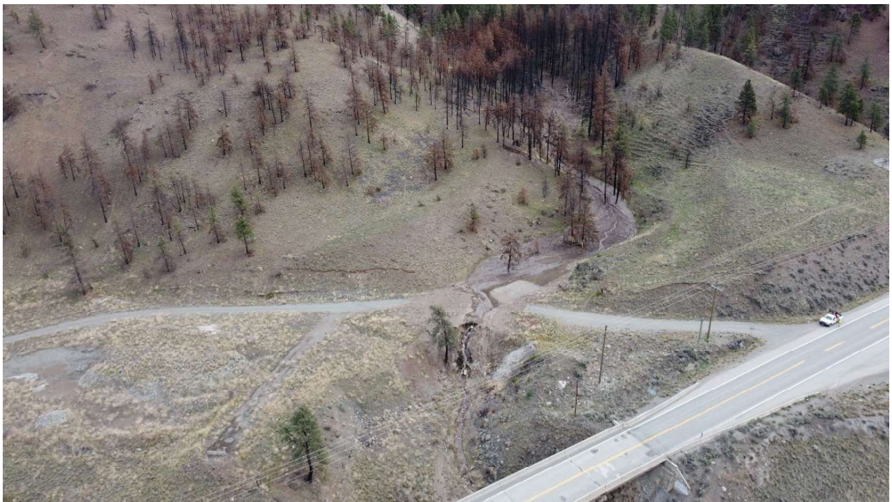
Figure 2.4 Approximate location of Sackum Creek crossing below the TCH, looking upstream
