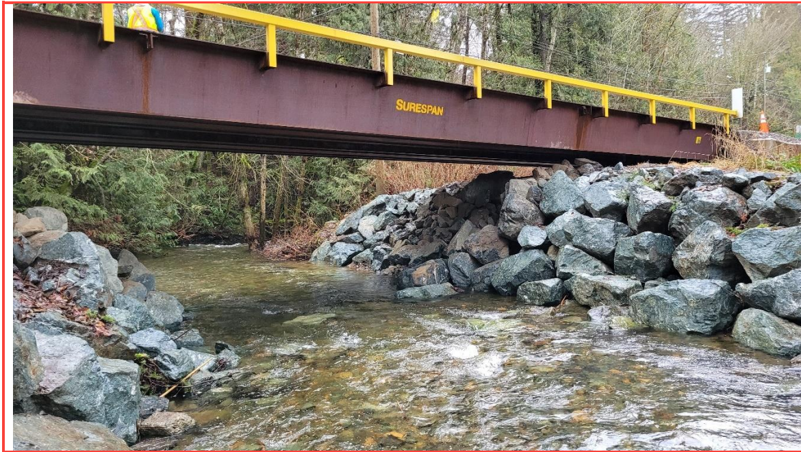
Photo: 9 Temporary repair condition looking towards the east bank.
