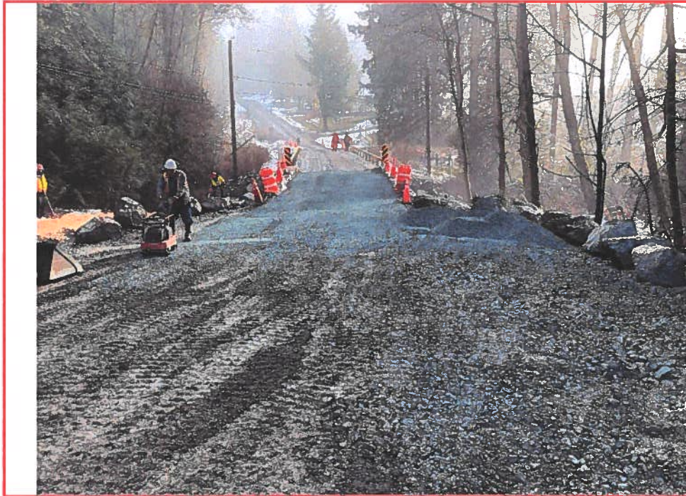
Photo 7: Overview of the NW side of the bridge Photo looking southeast.
