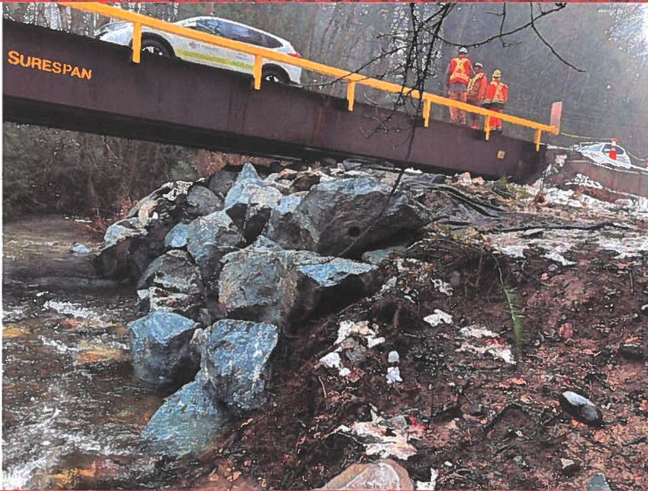
Photo 4: Looking northeast at the SE slope.
