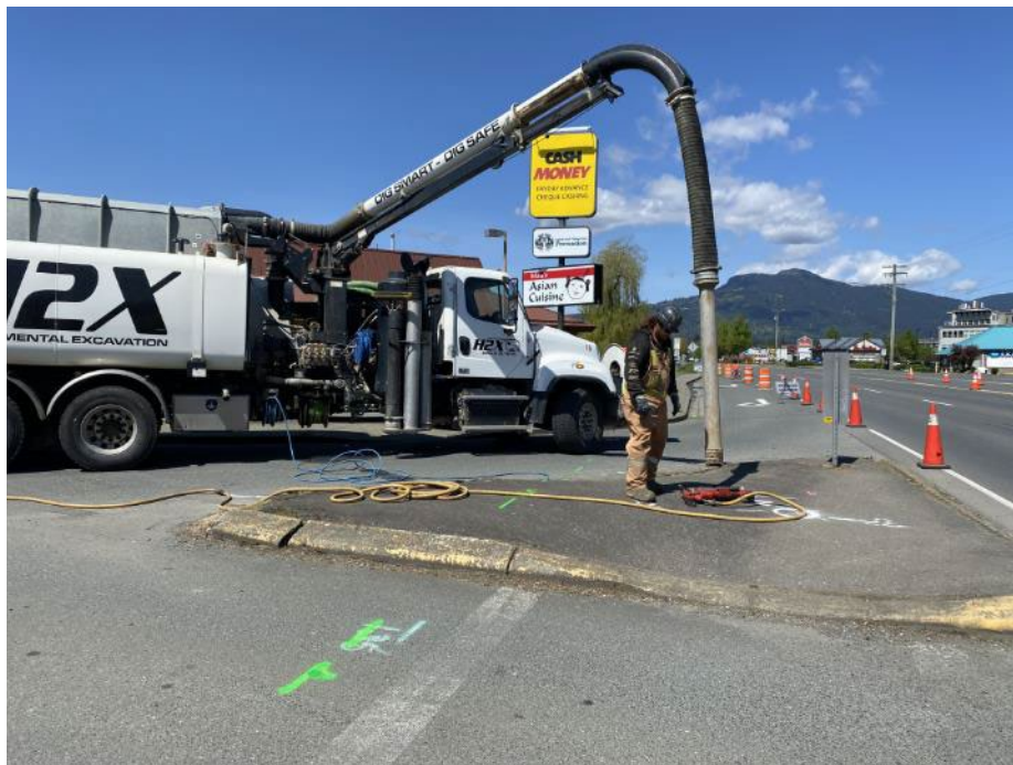
Photo 2: Advancing BH24-02 in traffic triangle using vacuum truck (May 8, 2024)
