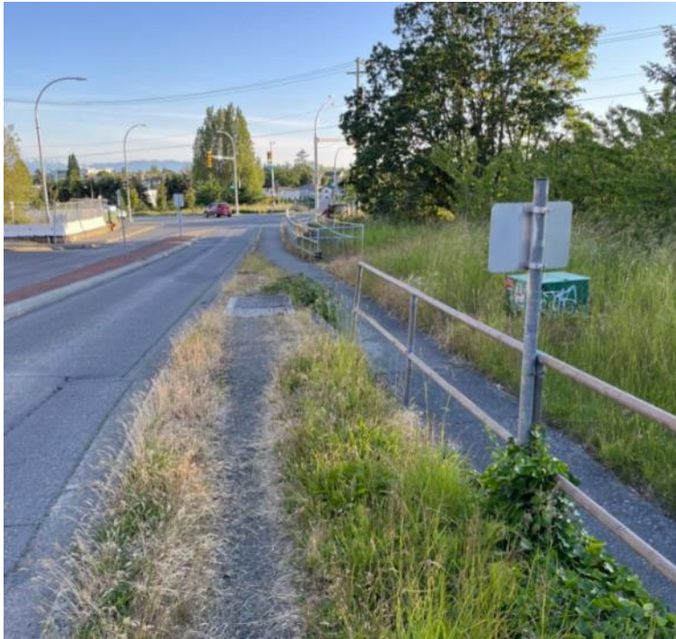
Photo 5: The Survey area south of Blanshard Street above the retaining wall. The grassy habitat is visible on the right side of this image. Photo facing southwest.
