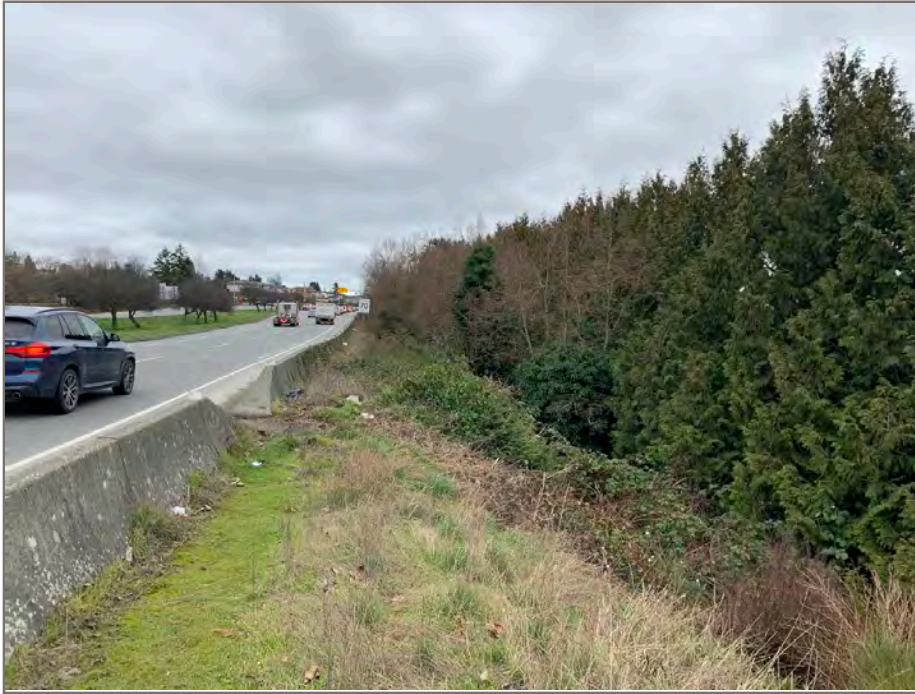
Photo 21: View of south-bound shoulder, east of Colquitz River Bridge (Area 6).
