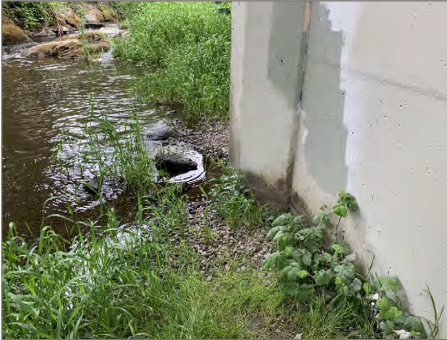
Photo 3: View looking upstream from below north-bound bridge (Bridge 01378). Bent #3 to the right in the photo was constructed below the high-water mark of the river.
