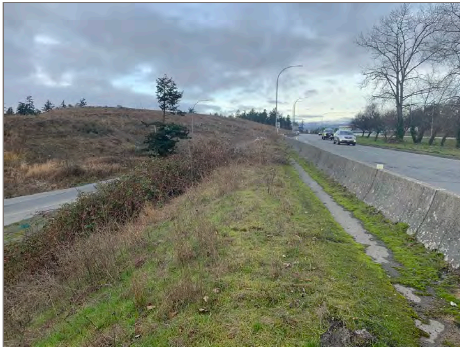
Photo 18: View of south-bound shoulder, west of Colquitz River Bridge (Area 3).
