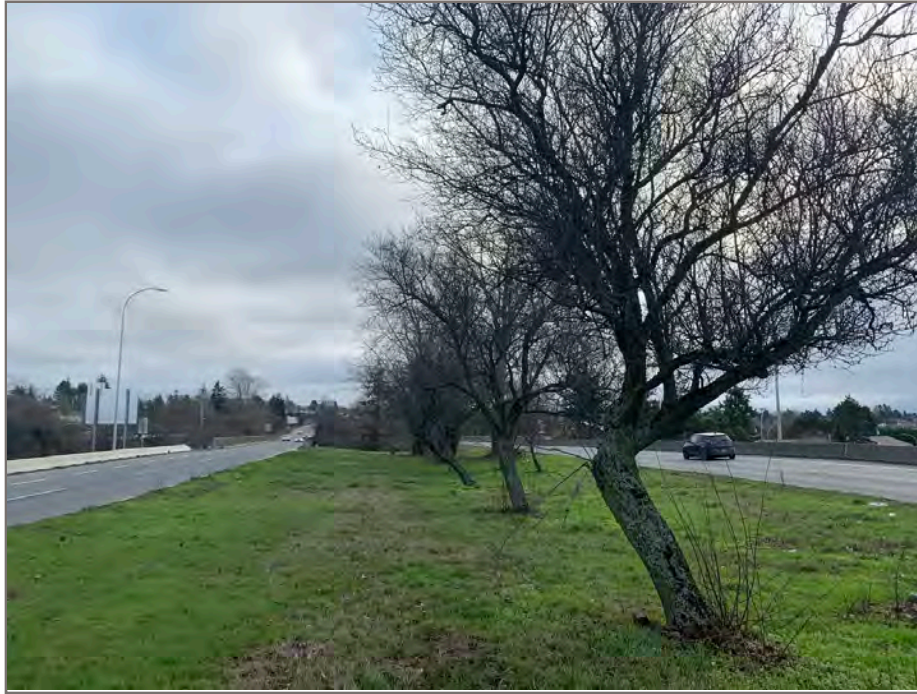
Photo 17: View of centre median, west of Colquitz River Bridges (Area 2).
