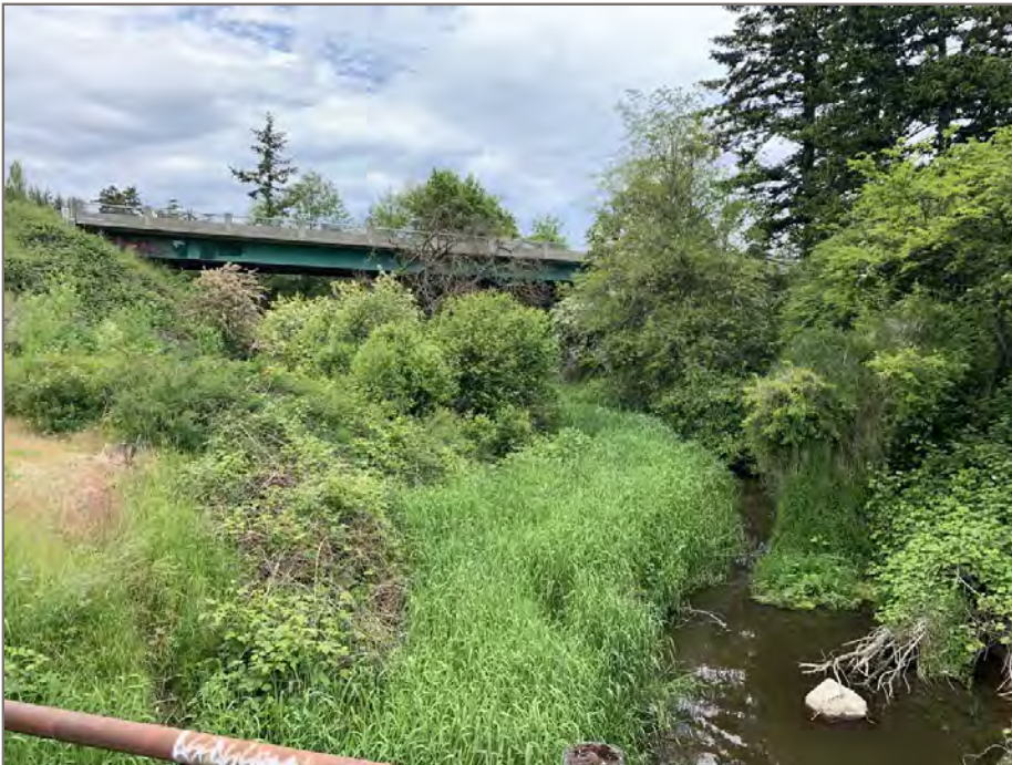
Photo 8: View upstream toward the south-bound bridge from the Highway 1 offramp onto Burnside Road - potential riparian enhancement area.
