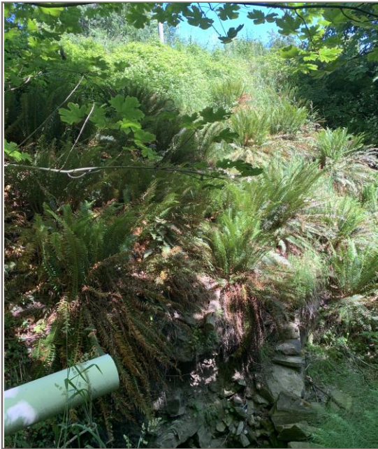
Photo 1: Looking southeast. View of the slope on west side of culvert/road
