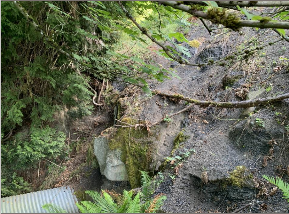
Photo 4: Looking south. View of the slope on east side of culvert/road
