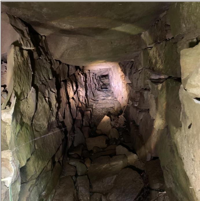
Photo 3: Looking east. View inside of stone cut culvert
