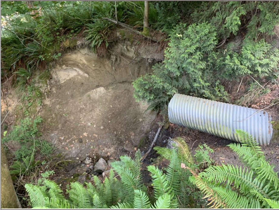
Photo 5: Looking east. View of the incised till-like soil near tow of slope on east side of culvert/road
