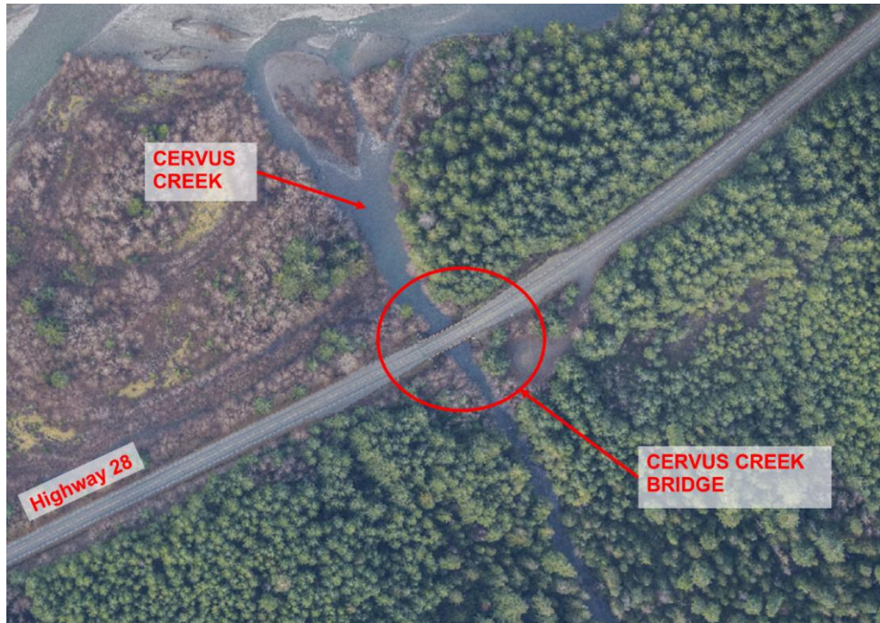
Figure 2-2 Cervus Creek Bridge Location (Source Google Map)
