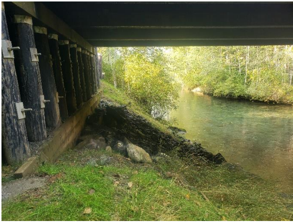
Photo 3: Cervus Creek looking north along west bank under existing bridge.
