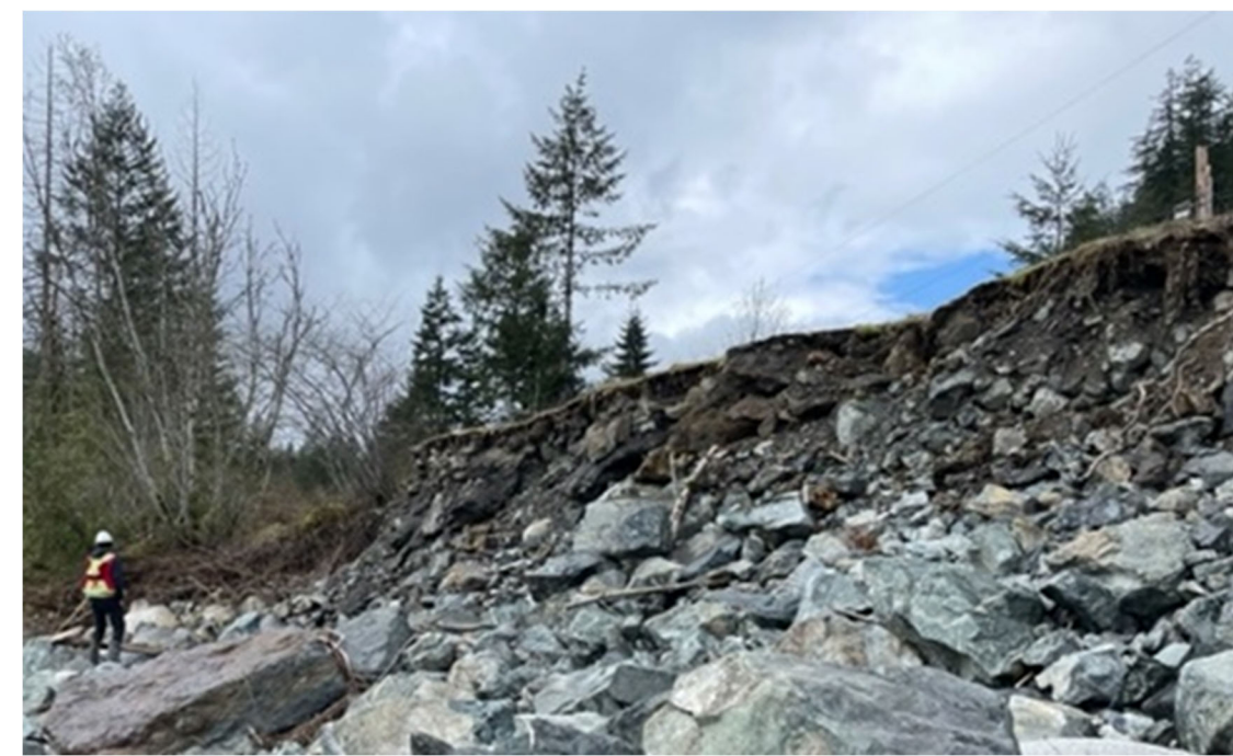
Figure 2-2 Photos of exposed bank slope and suspected embankment fill prior to construction of temporary riprap bank protection (March 31, 2022). (Left) Looking south at riprap and road base. (Right) Looking west upslope at road base and large riprap that remain in place.
