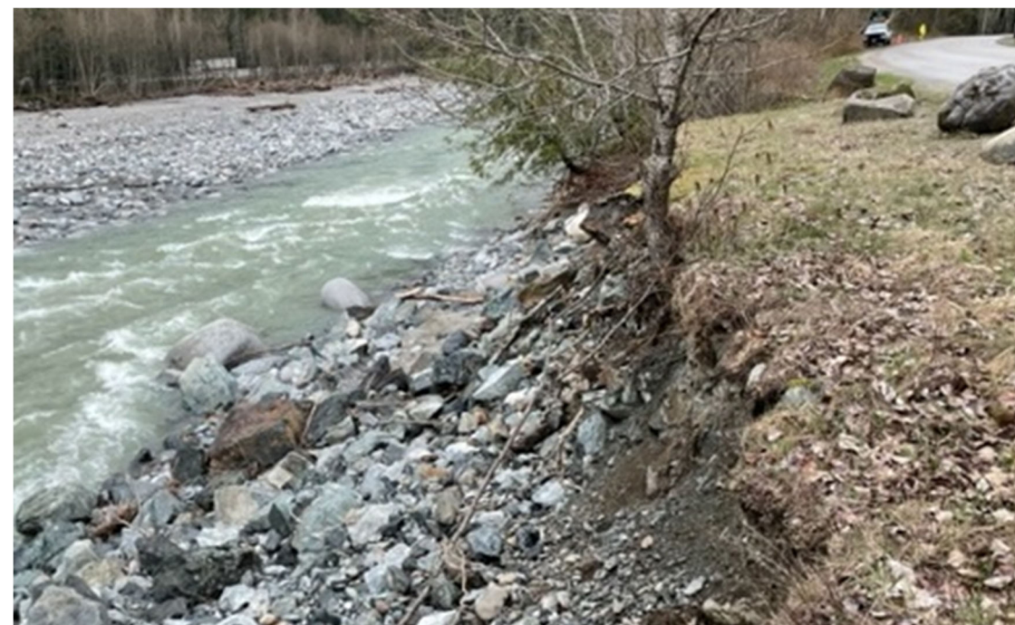
Figure 2-2 Photos of exposed bank slope and suspected embankment fill prior to construction of temporary riprap bank protection (March 31, 2022). (Left) Looking south at riprap and road base. (Right) Looking west upslope at road base and large riprap that remain in place.
