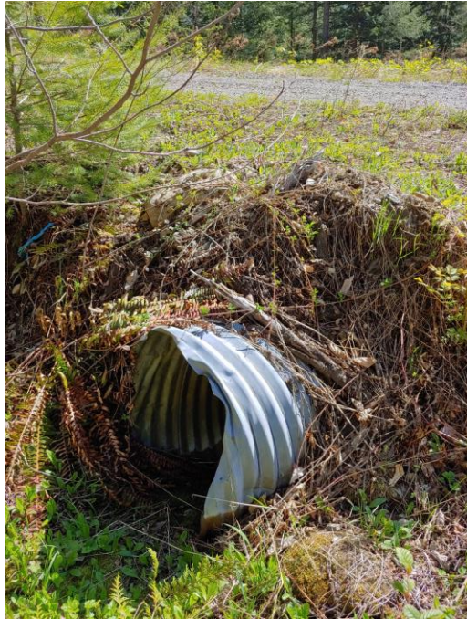
Photo 2-9: Ditch 1 Crossing Inlet, Northeast View
