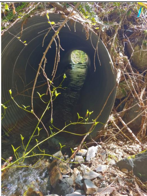
Photo 2-22: South Crossing Culvert Inlet and Embankment, Southeast View
