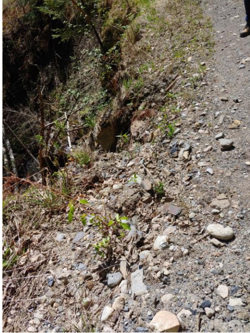
Photo 2-24: Outlet Embankment on the Southeast Side of the South Channel Crossing
