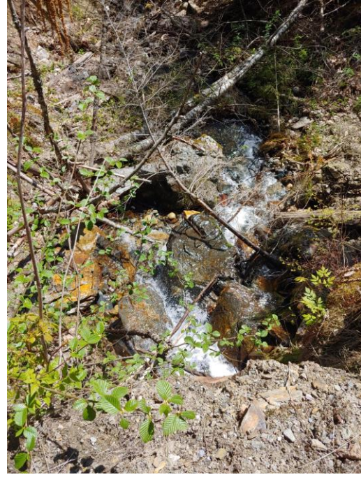
Photo 2-25: Outlet and Downstream of South Channel Crossing, Southeast View
