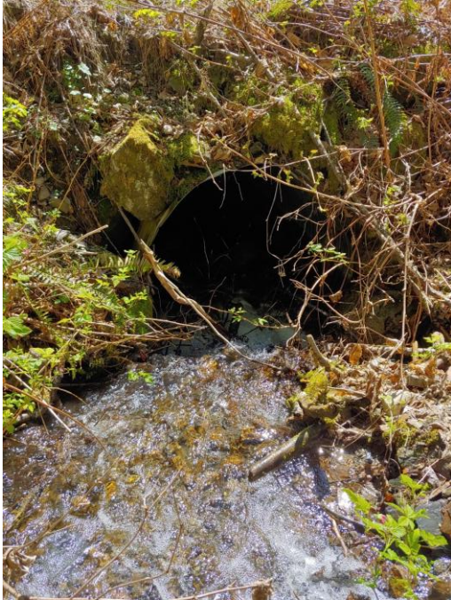
Photo 2-3: North Channel Crossing Inlet, East View
