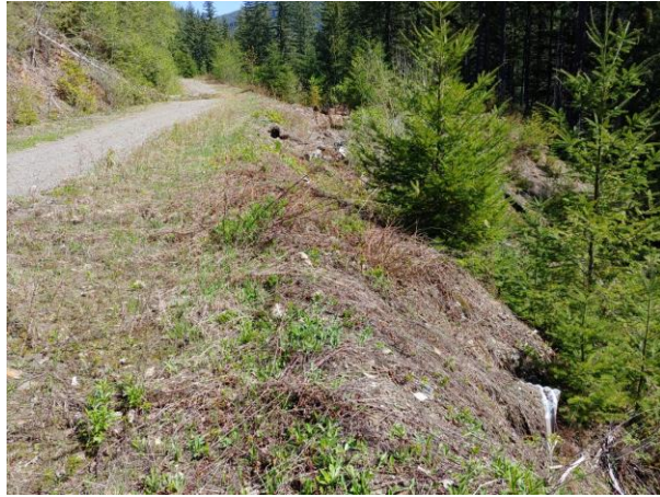
Photo 2-12: Roadway and Shoulder at Ditch 1 Culvert Outlet, North View
