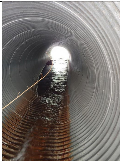
Photo 2-23: South Crossing Inside of Culvert, Southeast View from Inlet
