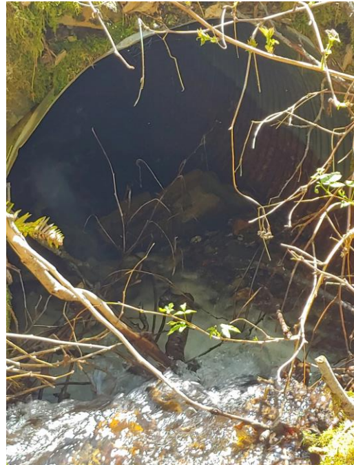
Photo 2-4: North Channel Crossing Inlet, East View
