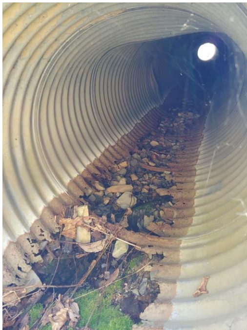
Photo 2-11: Ditch 1 Culvert, East View from Inlet
