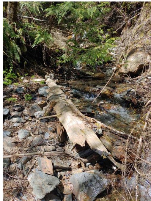
Photo 2-21: Channel Upstream of South Crossing, Northwest View
