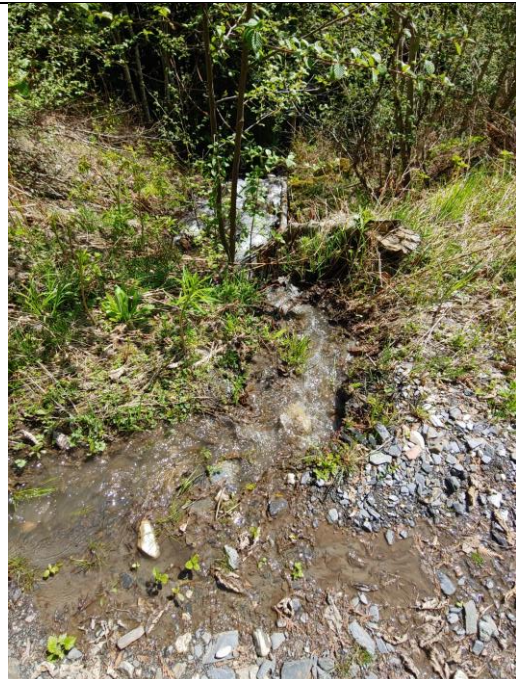
Photo 2-6: Water Flow on Road Turning East and Flowing Overtop of the North Crossing Outlet, East View
