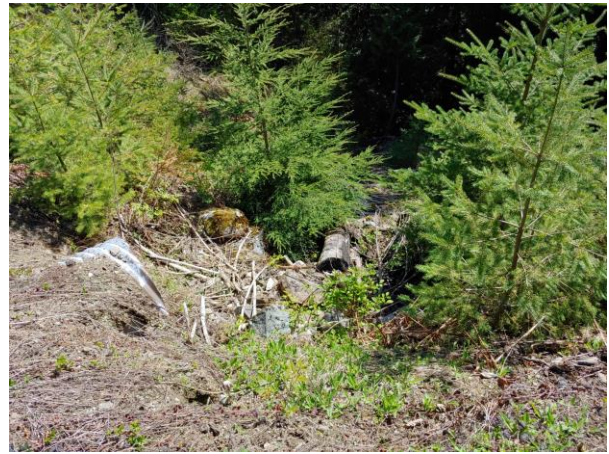
Photo 2-13: Channel Downstream from Ditch 1 Culvert Outlet, Northeast View
