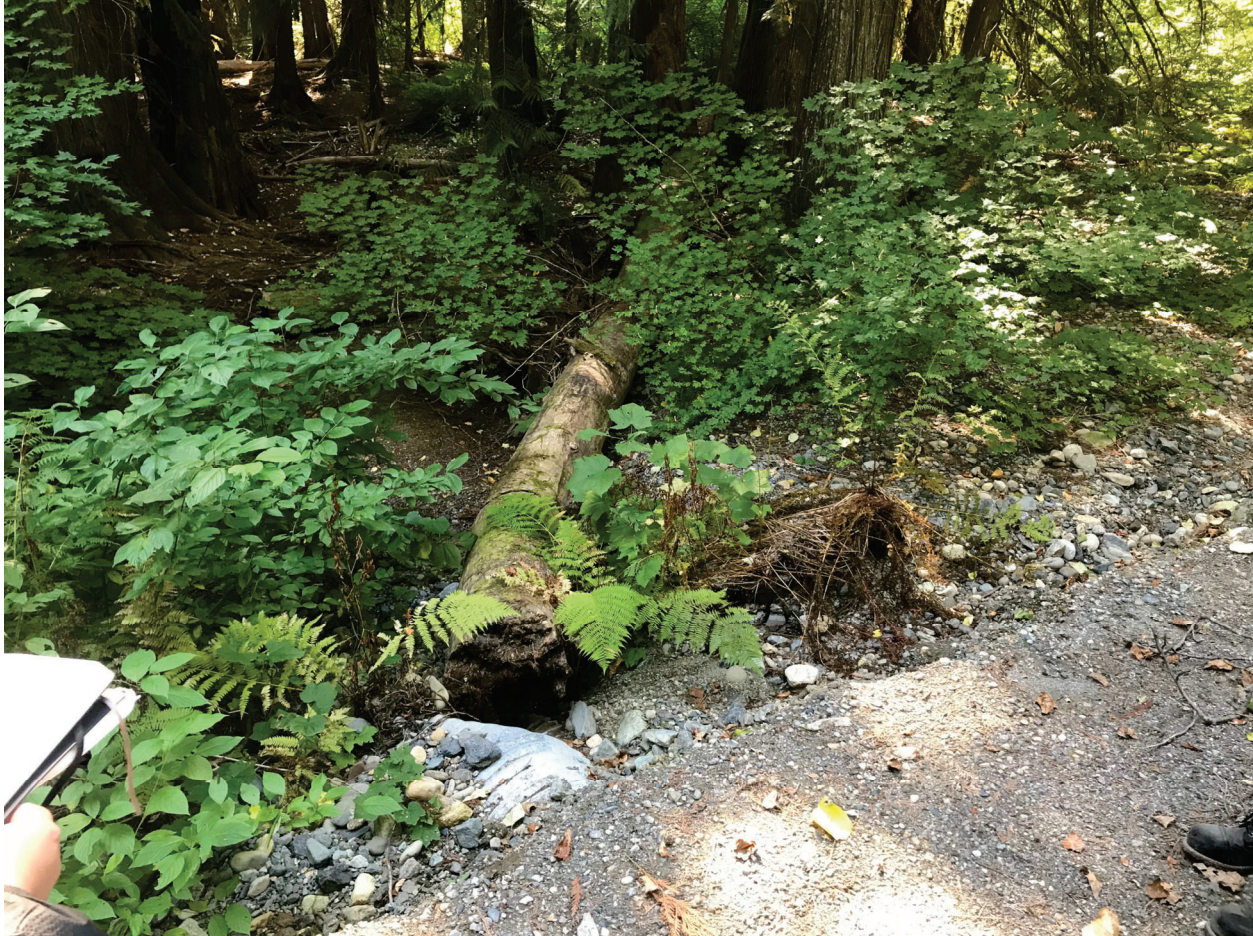
Photo 6: Culvert outlet near km 43.1, September 21, 2022
