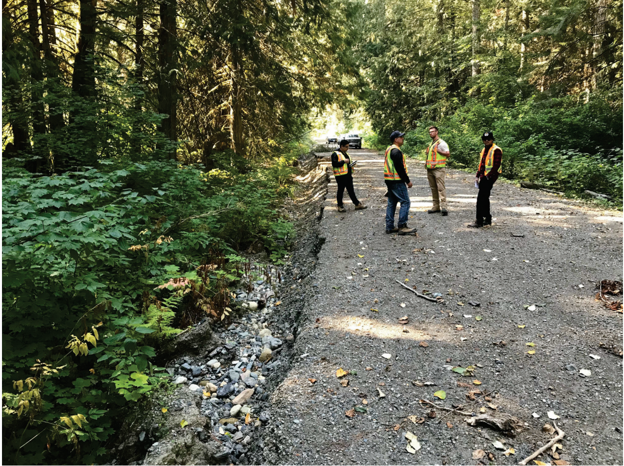
Photo 5: Looking north at the road at km 43.1, September 21, 2022. Note the erosion of the west shoulder.
