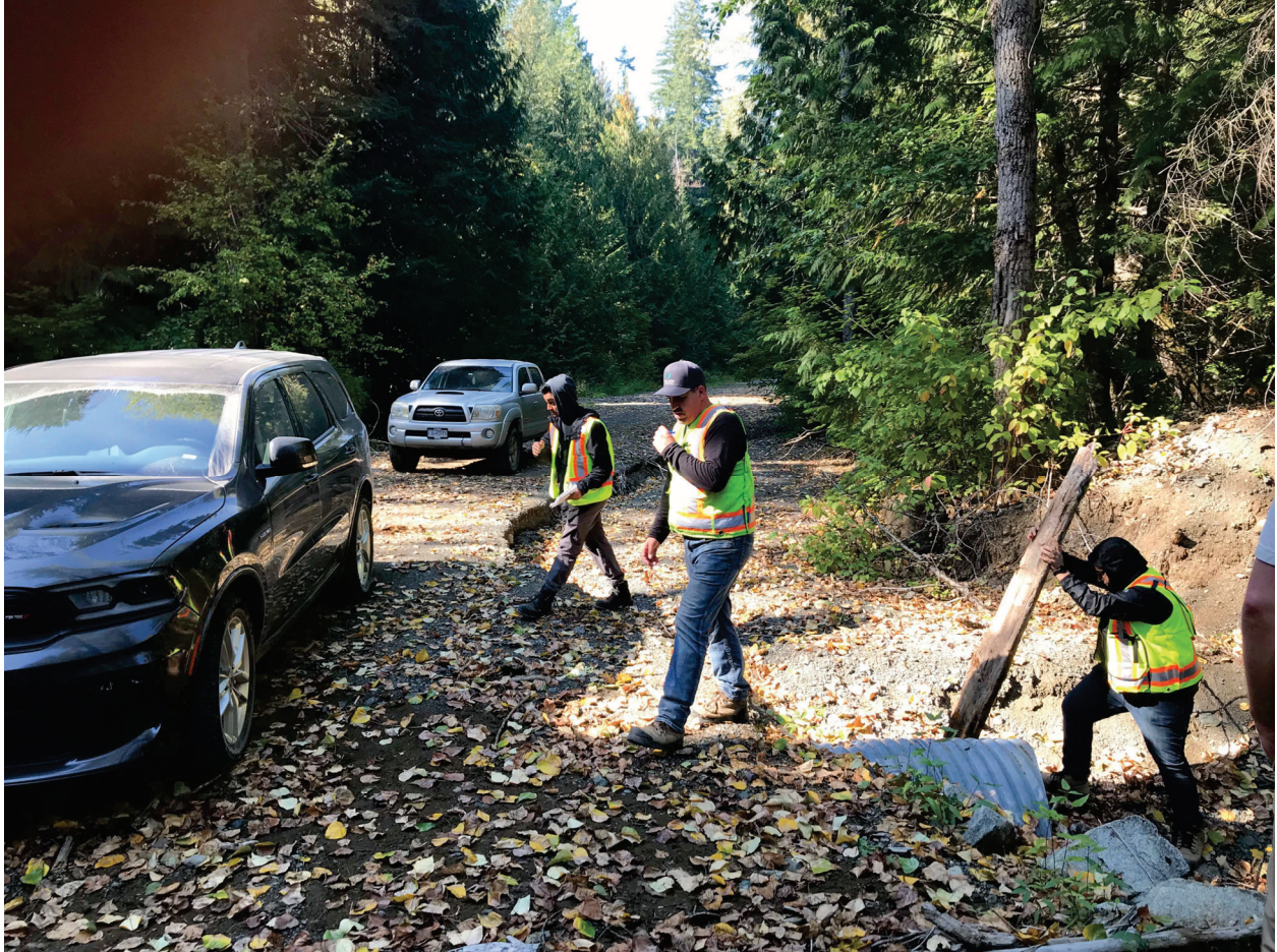
Photo 9: September 21, 2022. Looking north at culvert inlets at km 56.7. Note erosion along the east side of the road north of the creek channel.
