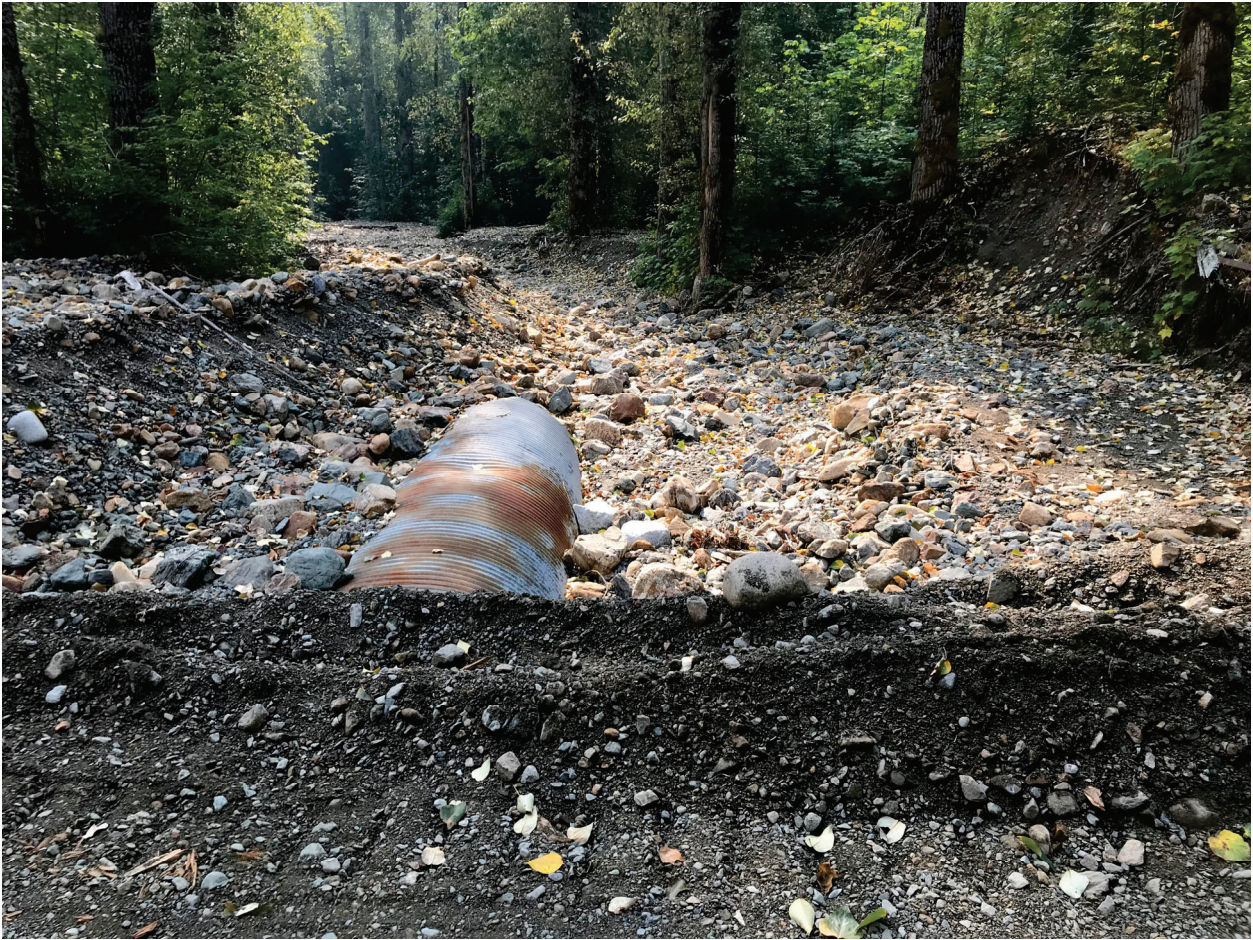
Photo 2: September 14, 2022. Looking downstream from the road.
