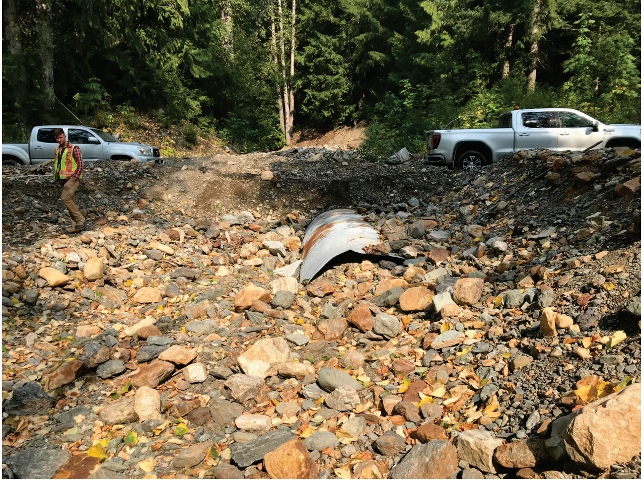
Photo 3: September 14, 2022. Looking upstream at the existing culvert outlet.
