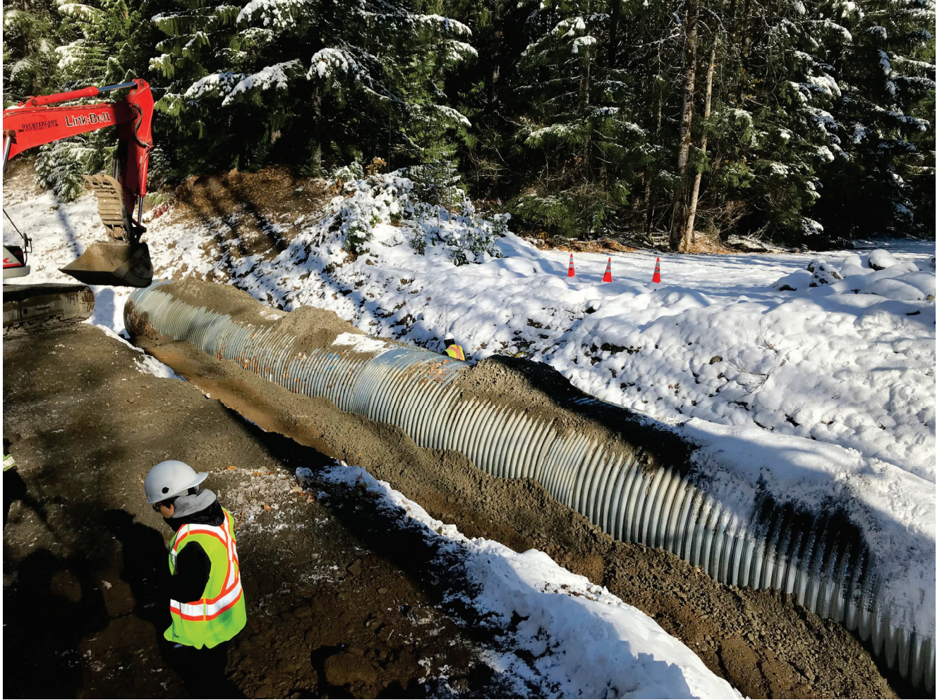
Photo 4: November 9, 2022; Culvert installation is in progress
