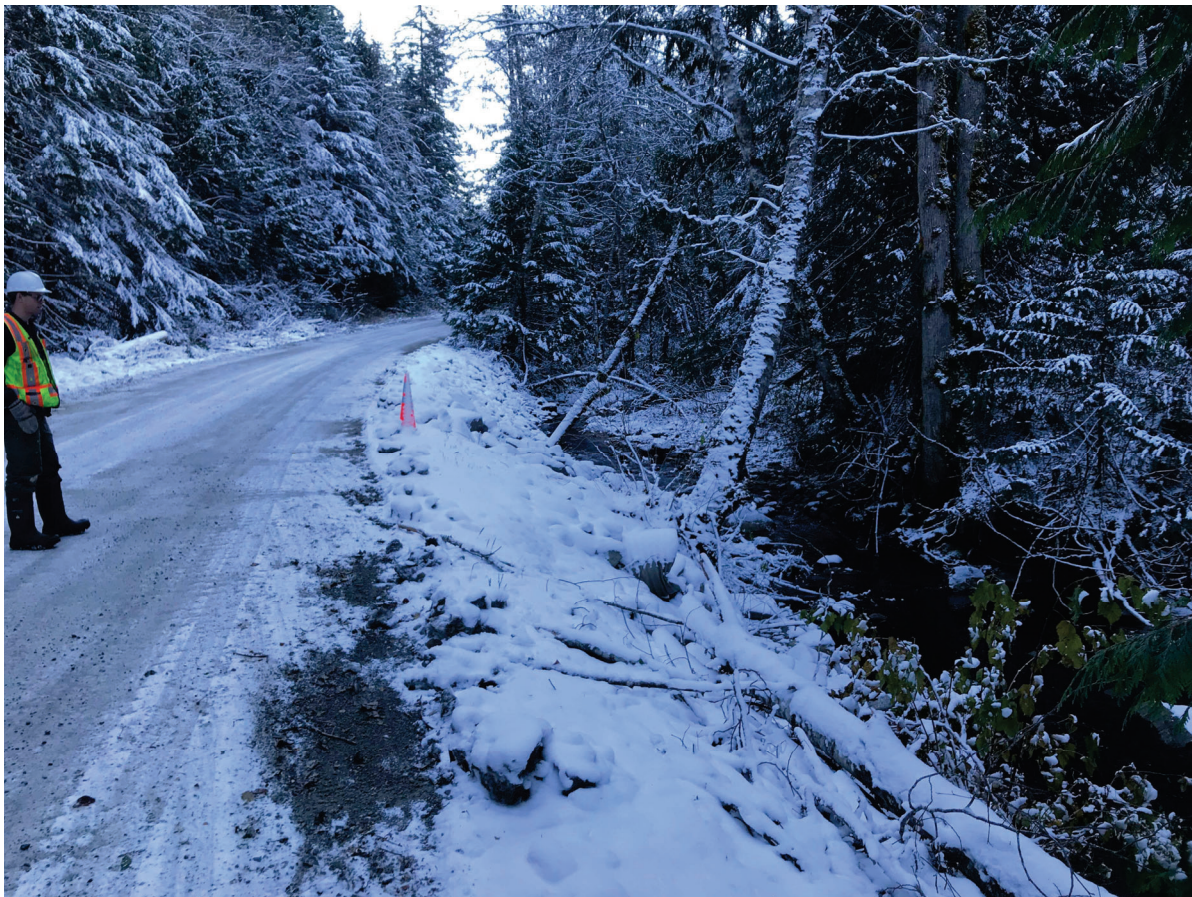
Photo 1: Looking south at the embankment on the west side of the road. Note the culvert outlet in the foreground.
