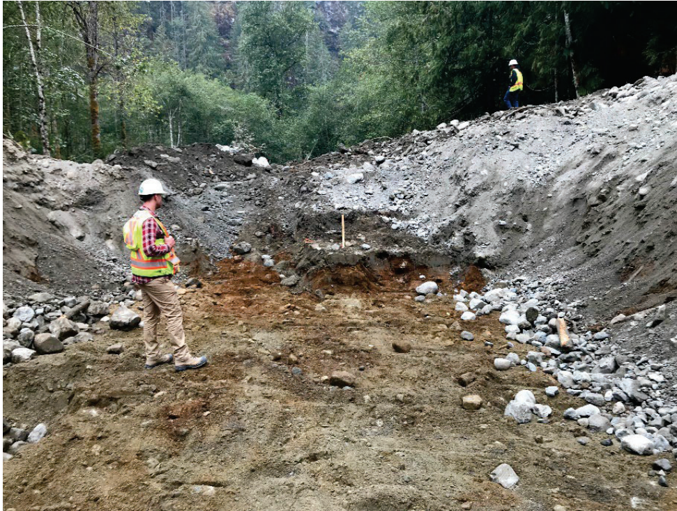
Photo 1: Looking west at the culvert excavation for the creek at km 10.9
