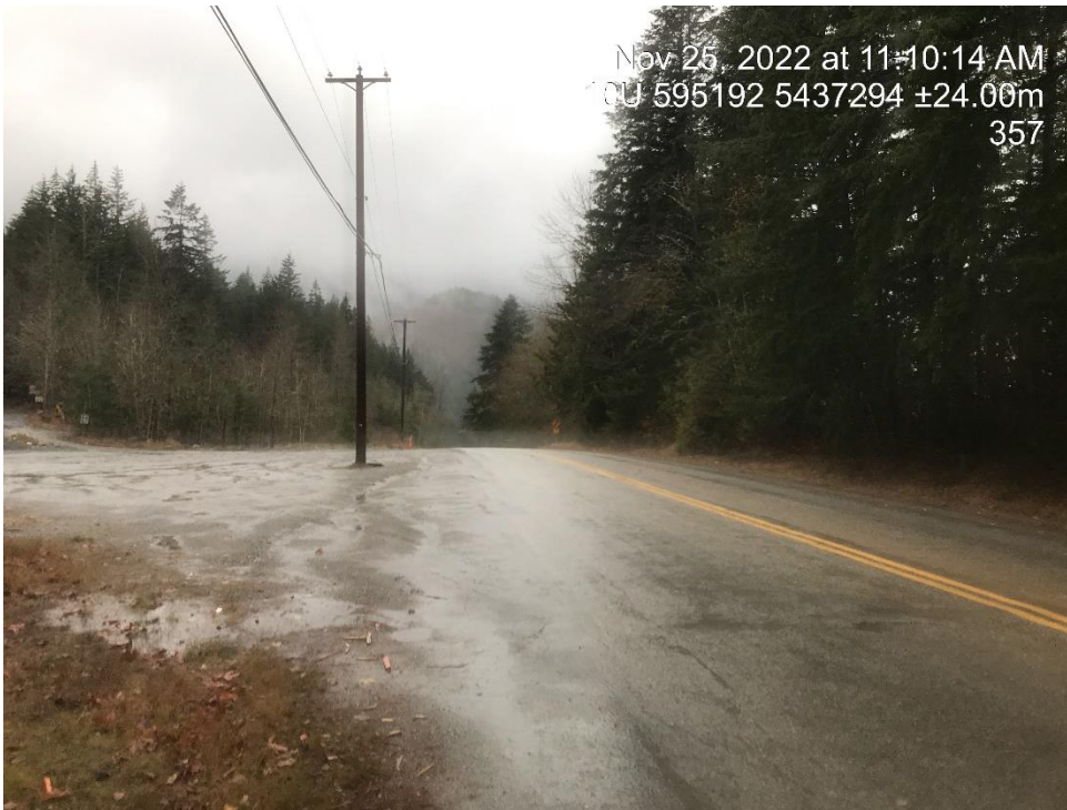
Photo 1: Eastern end of Project, looking west. 25 November 2022.
