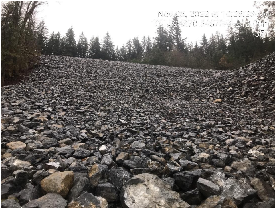
Photo 3: Stabilization of the slope failure area. 25 November 2022.
