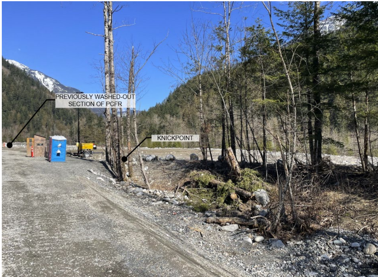
Figure 5-2. View of potential knickpoint immediately south of previously washed-out section of PCFR. Photo Source: BGC, March 21, 2023.
