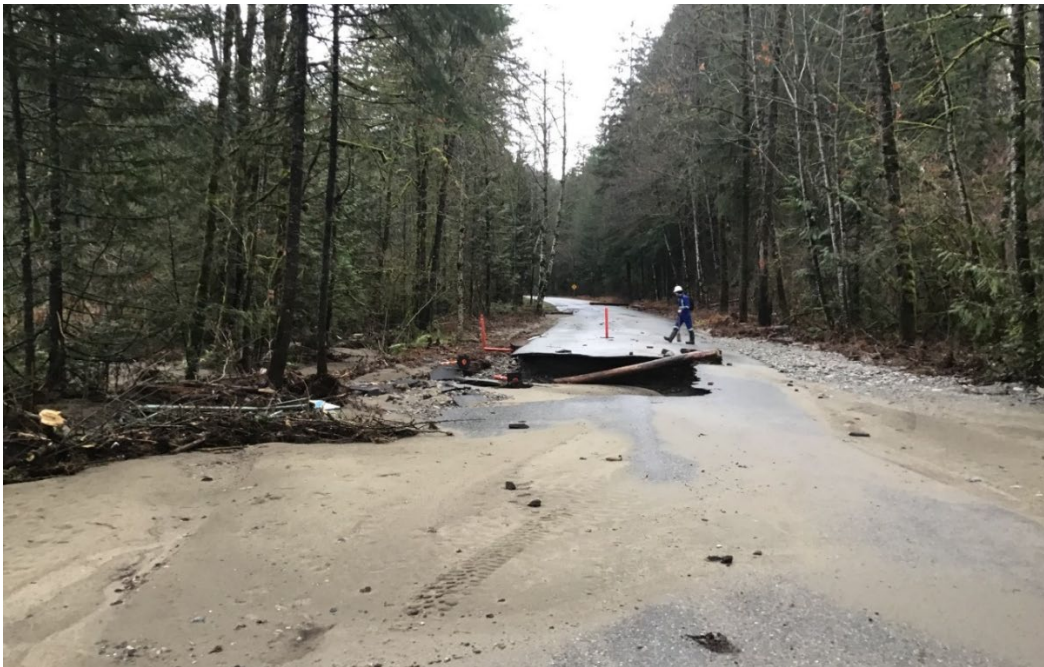
Figure 1-1. Example of a HWM from the Coquihalla River flooding. Sediment deposited along Othello Road is clearly visible. Photo: BGC, December 2, 2021.
