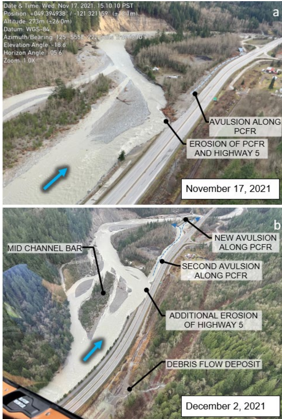
Figure 1-2. Photographs from a) November 17, 2021 and b) December 2, 2021 showing the erosion and avulsion at Peers Creek Frontage Road.
