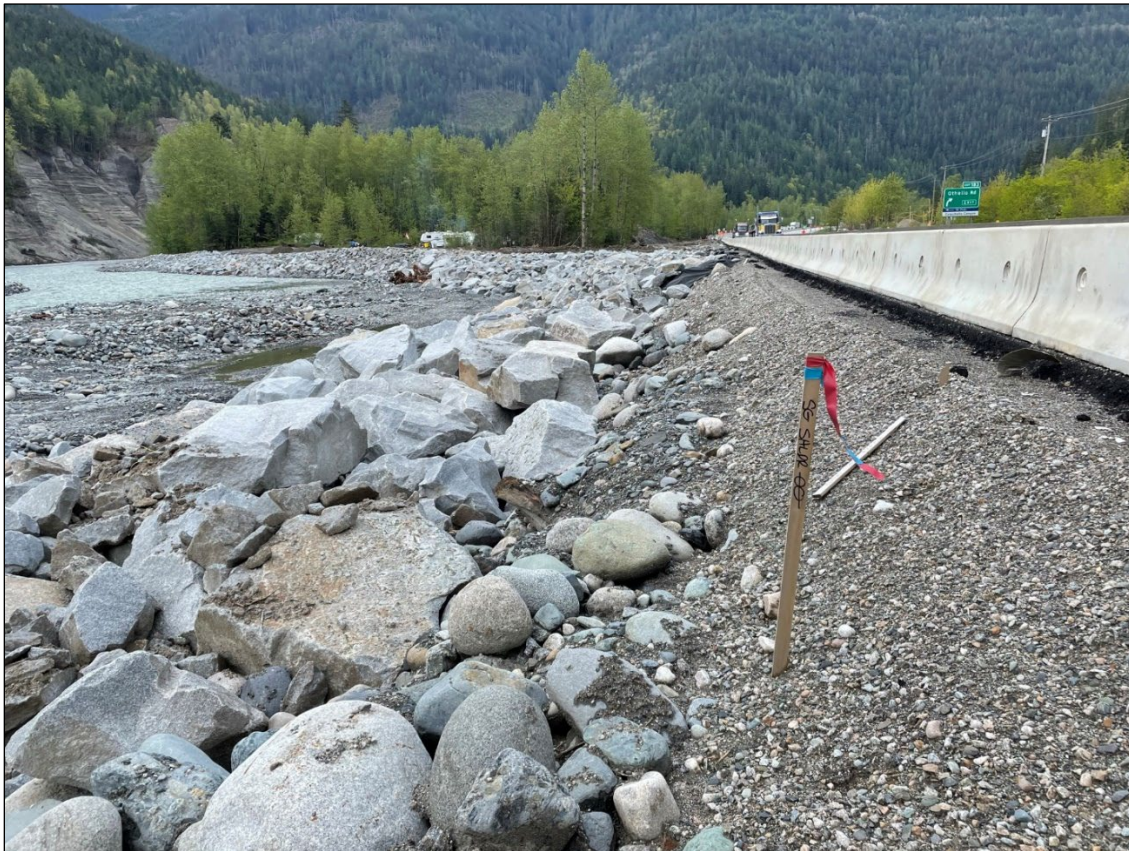
Figure 4-1. Looking downstream along emergency bank protection place on the right bank of the Coquihalla River. Photo Source: BGC, May 9, 2022
