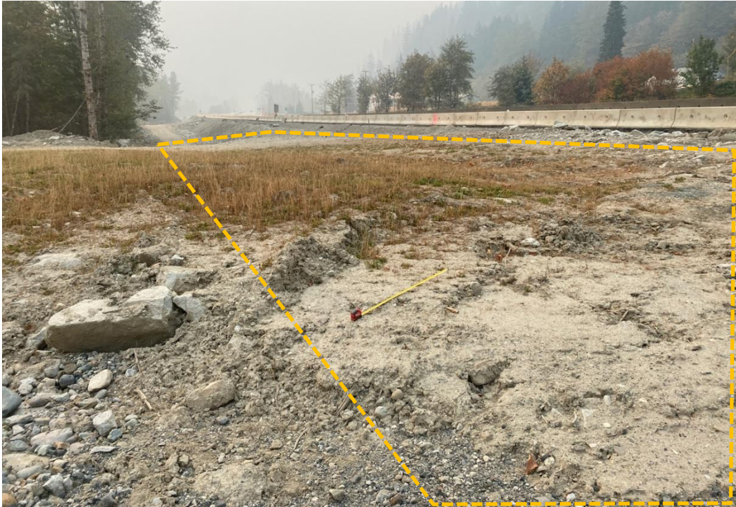
Photograph 9. View looking southwest (downstream) showing embankment fill (in orange) during the initial response work with the measuring tape extended to 1 m in the photo. Apparent topsoil layer was placed on the embankment fill and seeded (Photograph by BGC taken on October 18, 2022).
