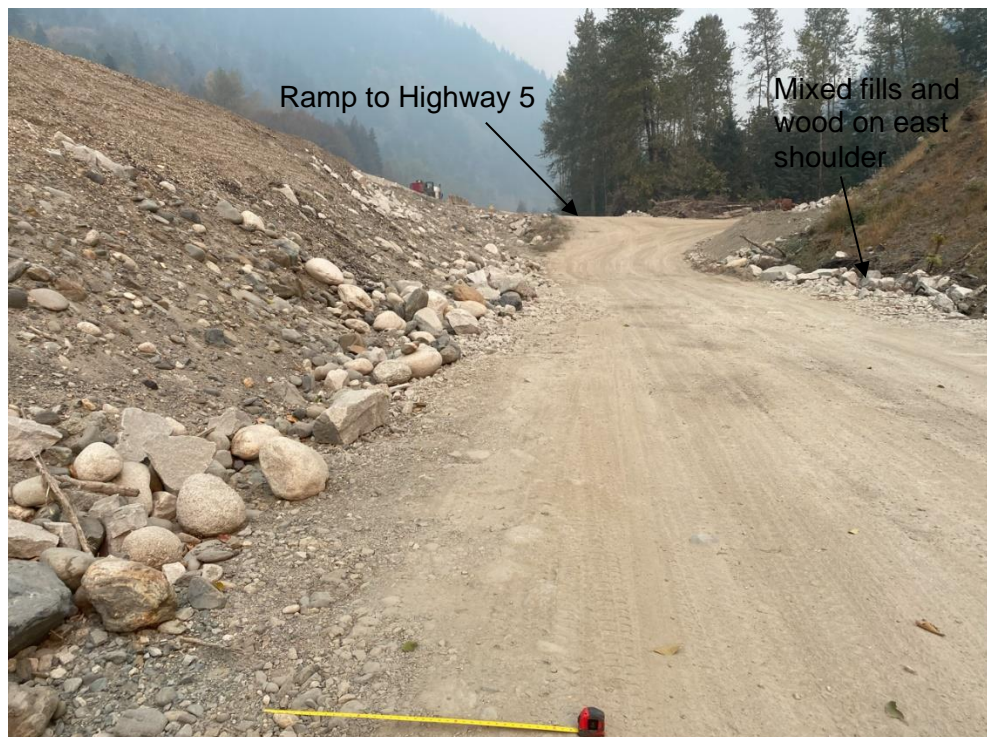
Photograph 12. View looking north (upstream) along the previous PCFR alignment at the fill placed early in the response phase of work, the measuring tape extended to 1 m in the photo (Photograph by BGC taken on October 18, 2022).
