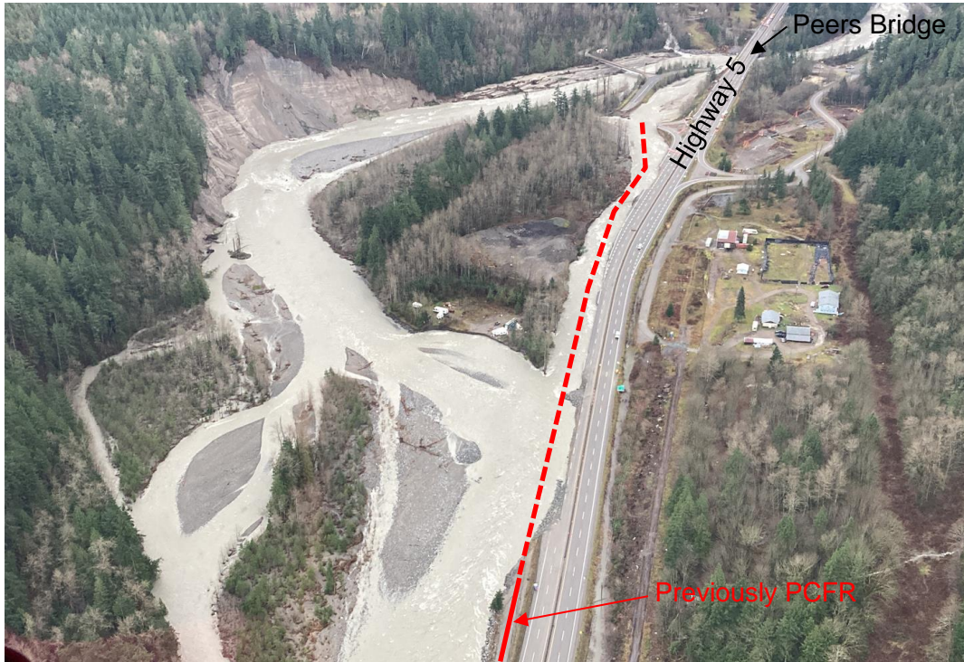
Photograph 1. Aerial view looking south (downstream) with the red dashed line showing the washout of the Peer's Creek Frontage Road (PCFR) which run adjacent to eastbound Highway 5 (Photograph provided by MoTI taken on December 2, 2021).
