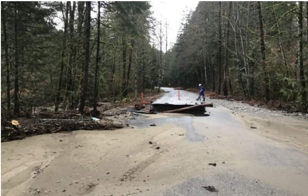
Figure 1-1. Example of a HWM from the Coquihalla River flooding. Sediment deposited along Othello Road is clearly visible. Photo: BGC, December 2, 2021.
