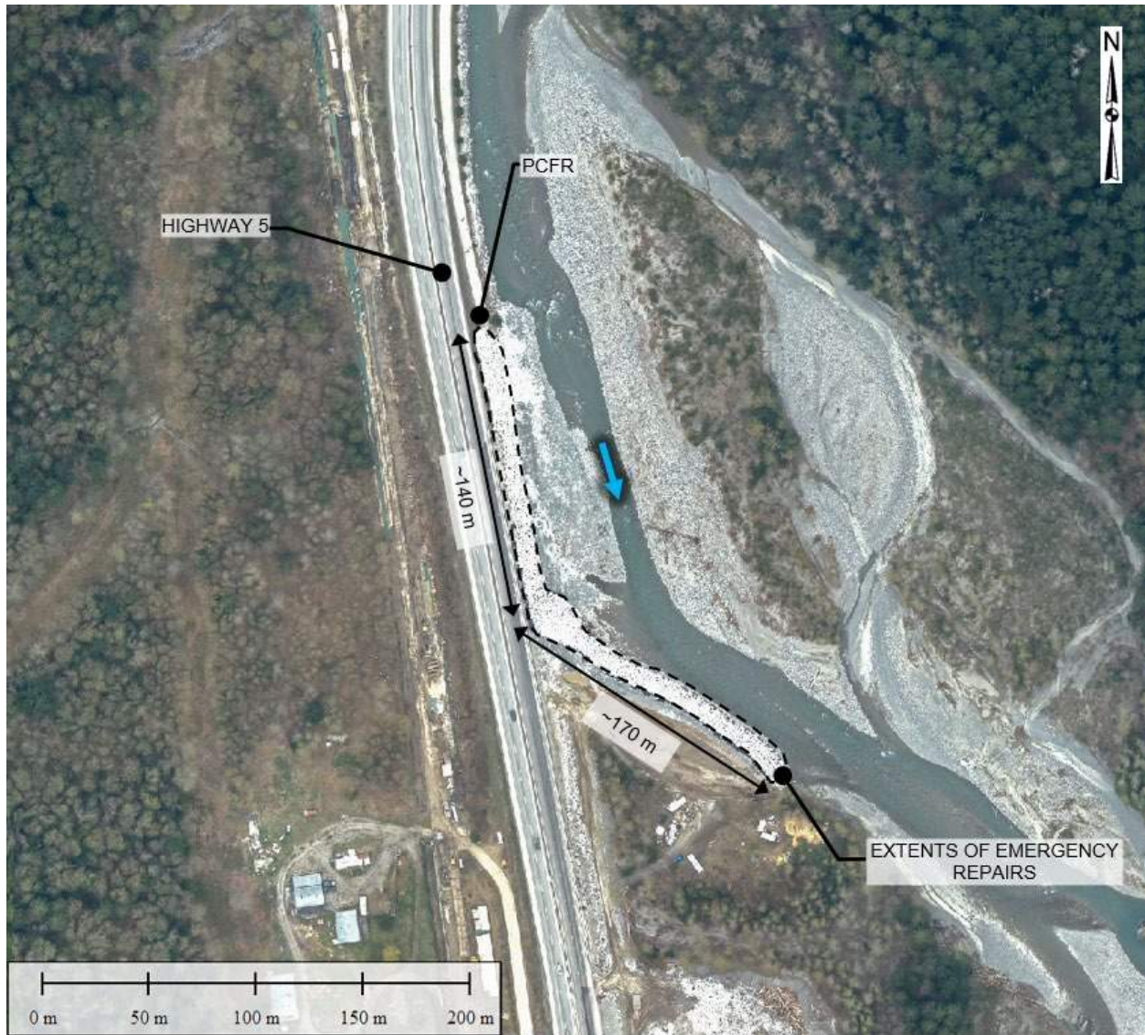
Figure 4-2. Overview of emergency repair extents along PCFR and Highway 5. Base Imagery Source: McElhanney, April 20, 2022
