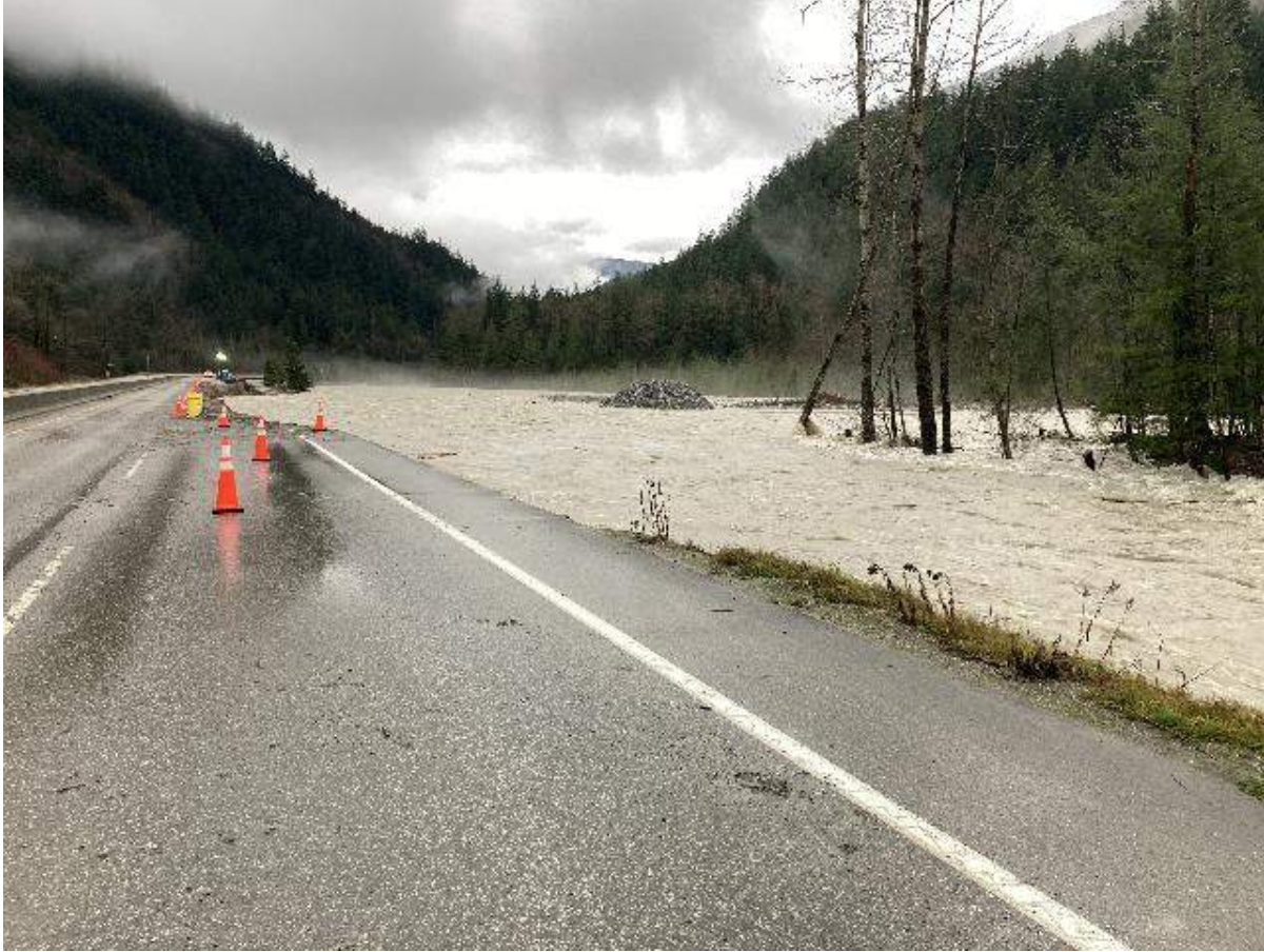
Photo 3. Looking north at flooding and washout area along Highway 5 in November 2021.
