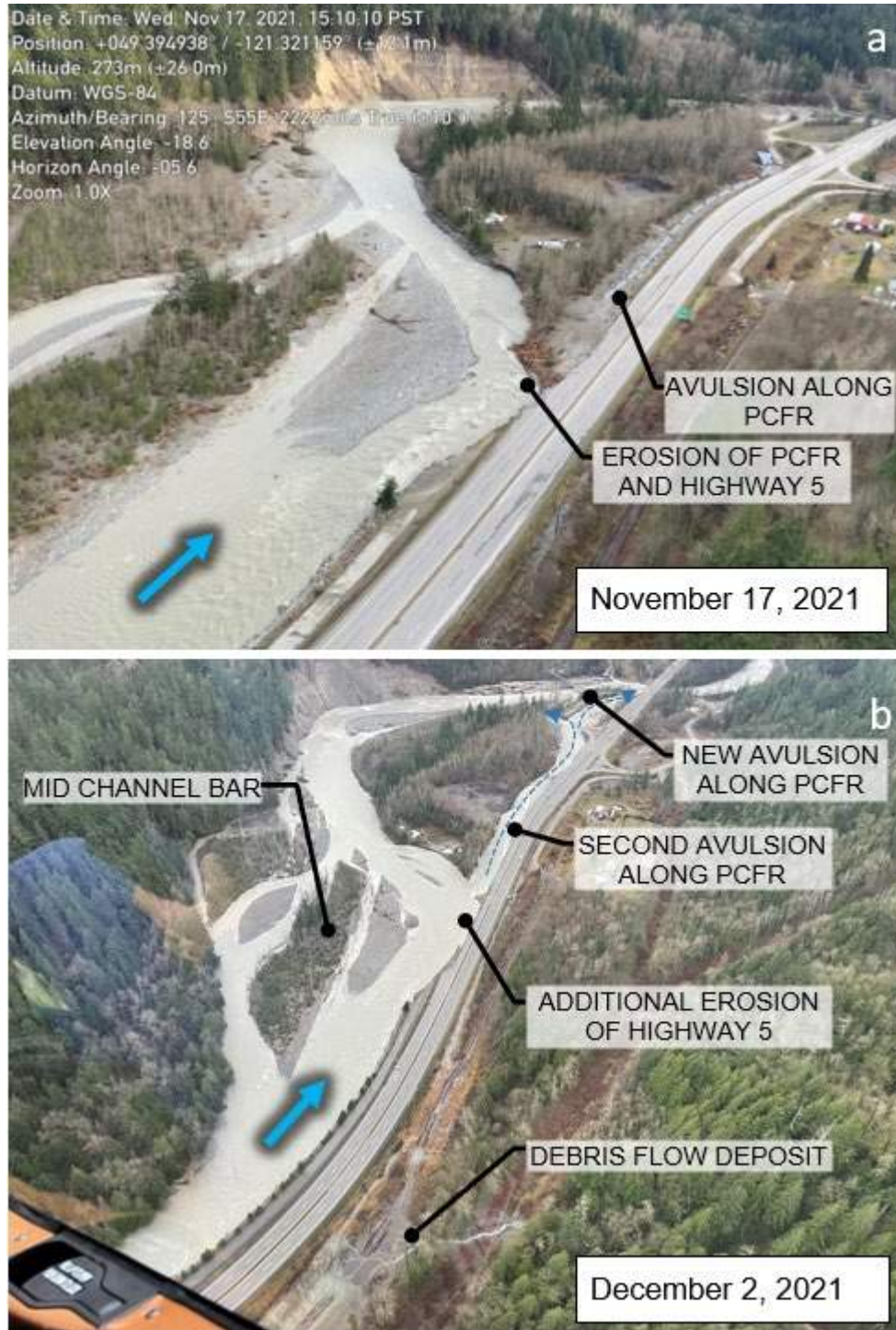
Figure 1-2. Photographs from a) November 17, 2021 and b) December 2, 2021 showing the erosion and avulsion at Peers Creek Frontage Road.
