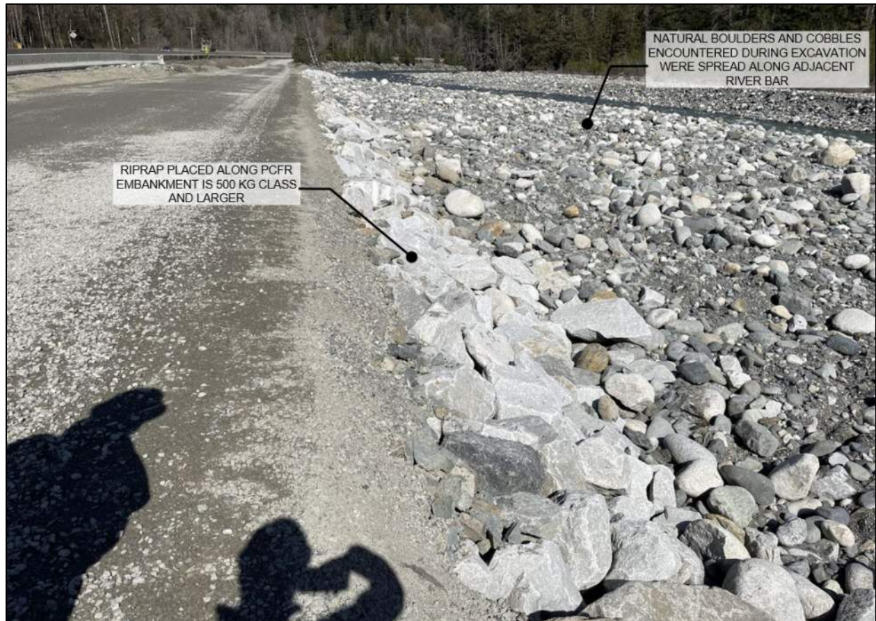
Figure 4-4. View of interim road repairs looking upstream (north). Photo Source: BGC, March 21, 2023.
