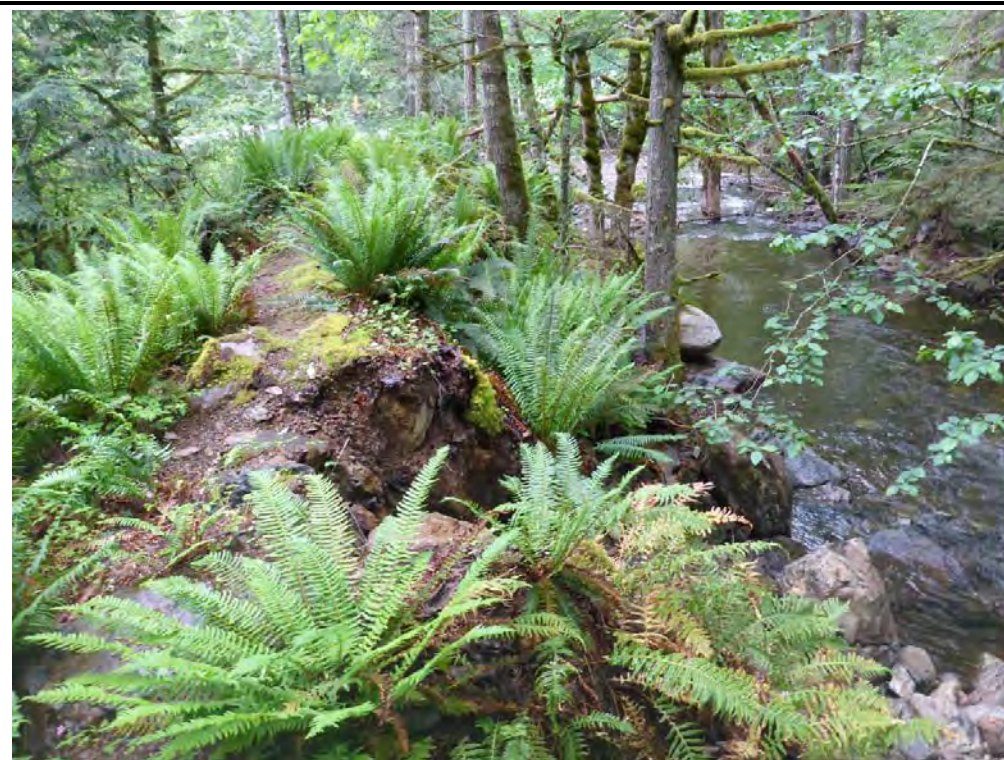
Photo 2 – Looking downstream Trout Lake Creek toward the Crossing. The man-made berm is visible in the foreground.
