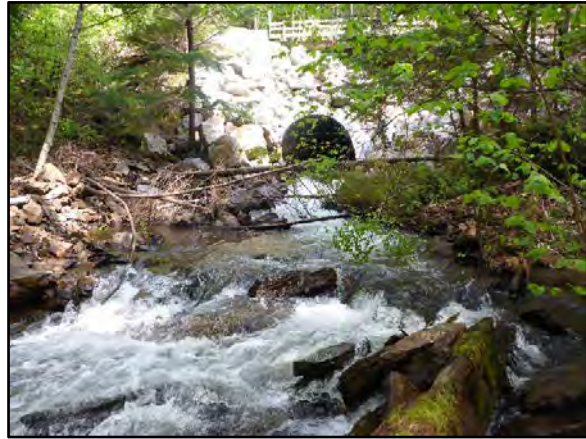
Riffle and cascade downstream of Rockwell Drive (upstream view).
