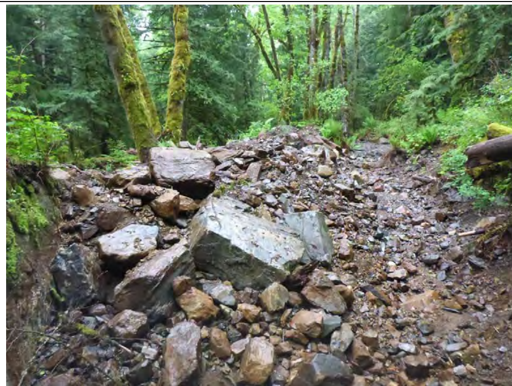
Photo 5 – Looking downstream (north) at the avulsion in Stream 1 near Wpt 035. The berm to the left has been repaired after the breach in February 2020.
