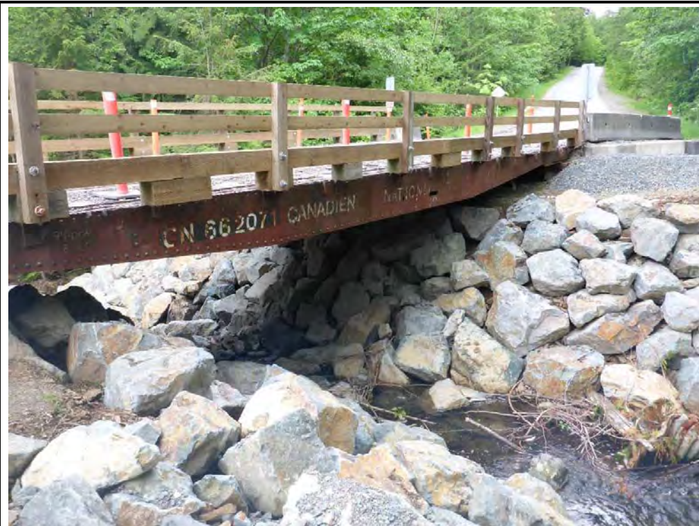
Photo 1 – View of the temporary crossing at Wpt 001.
