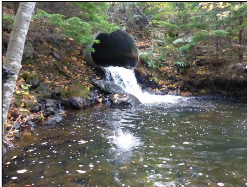
Figure 5 Rockwell Drive culvert outlet (November 8, 2017).
