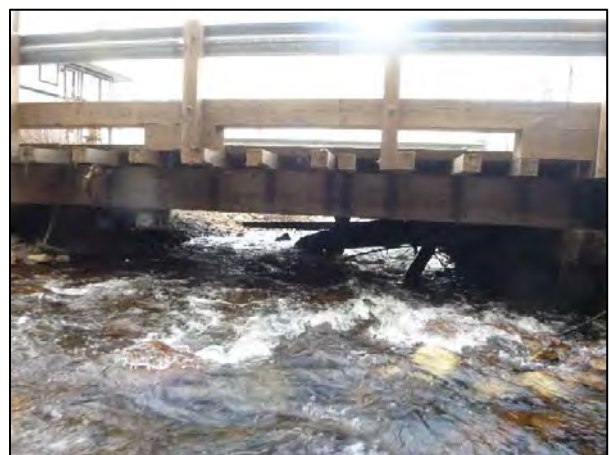
Photo 2 Downstream (west) view showing post-flood clearance under Green Point Bridge. (March 30, 2022).
