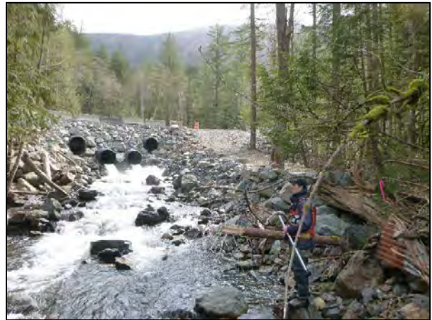
Photo 6 Trout Lake Creek downstream of Hicks Lake Road. (upstream view; March 30, 2022).
