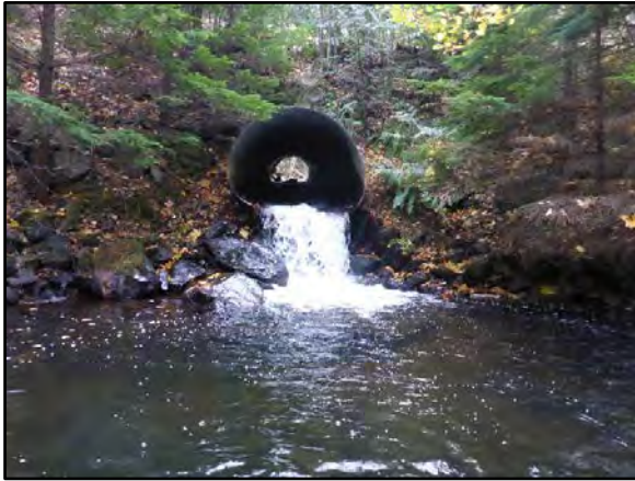
Plunge-pool downstream of Rockwell Drive (upstream view).
