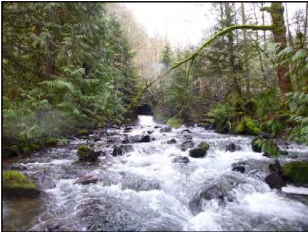
Photo 5 Trout Lake Creek downstream of Hicks Lake Road. (upstream view; March 26, 2018).
