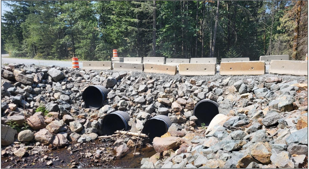
Photo 5. Sample image of the existing drainage DF#4 – above the road.
