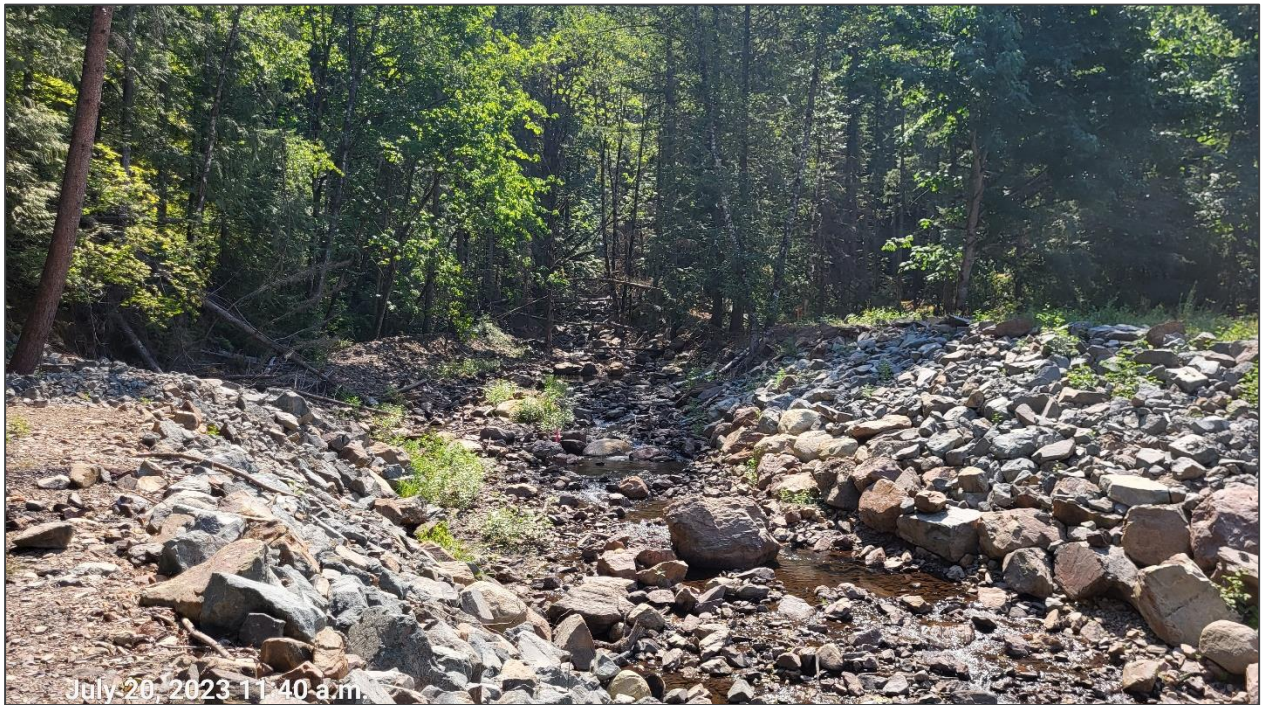
Photo 6. Sample Image of SF#4 – above the road.
