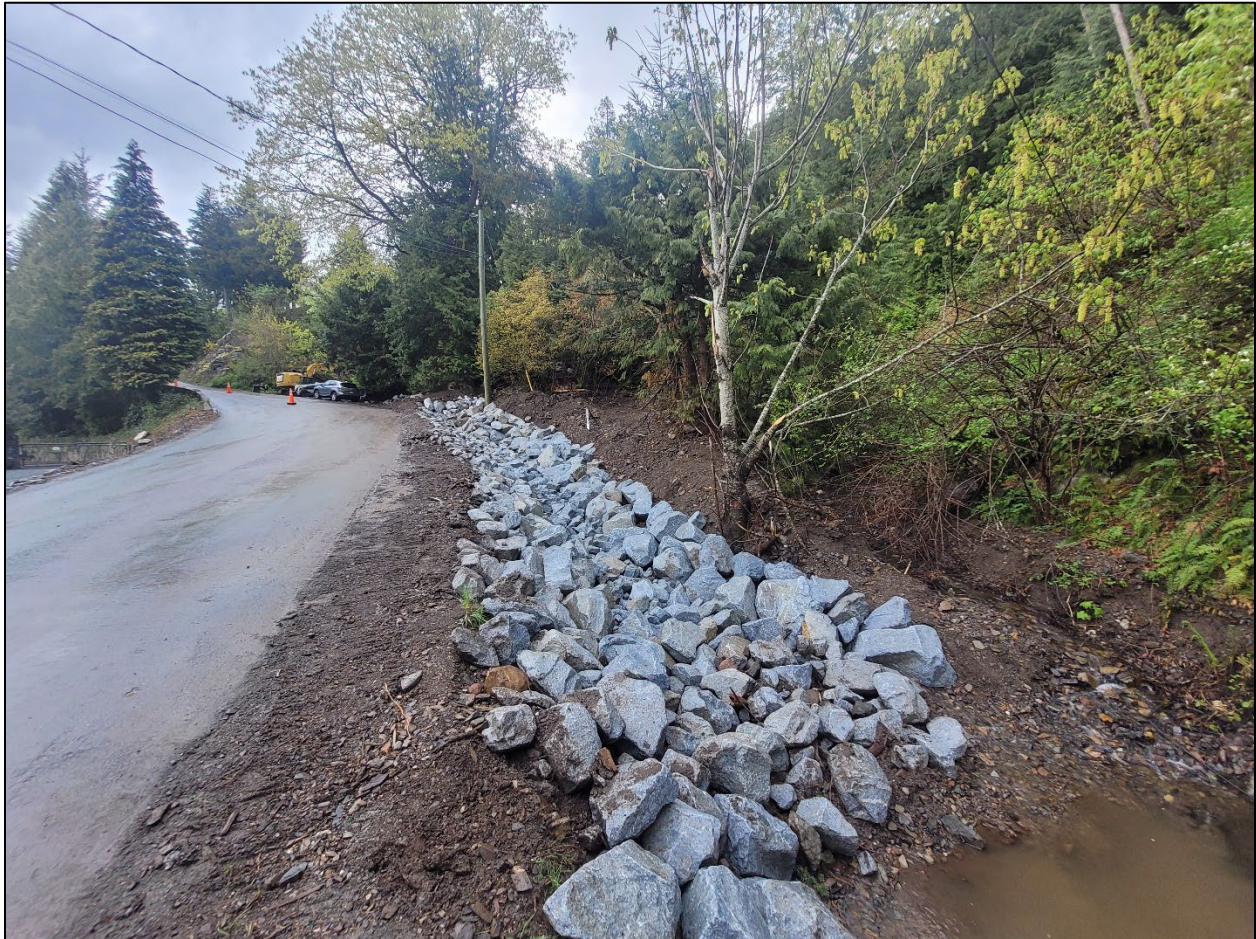
Figure 7 Short-term recovery works at site DF2 (April 26, 2022).
