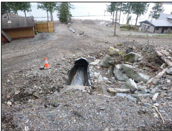
Photo 3: Downstream of Rockwell Drive the DF1 watercourse is culverted on private property.
