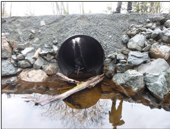
Photo 3: Rockwell Drive culvert inlet.
