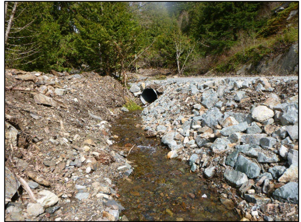
Photo 2: Upstream view of the Rockwell Drive culvert outlet.
