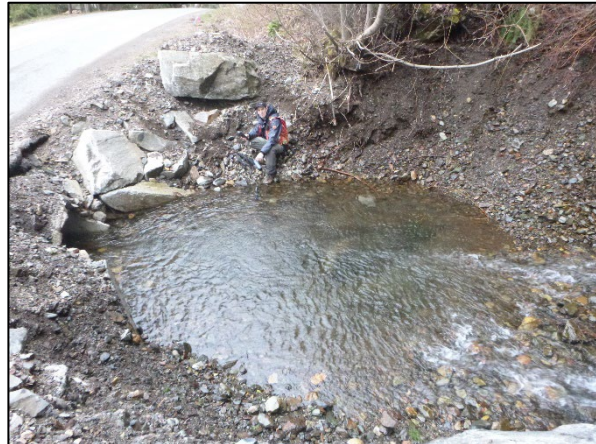
Photo 2: Large pool at the Rockwell Drive culvert inlet.
