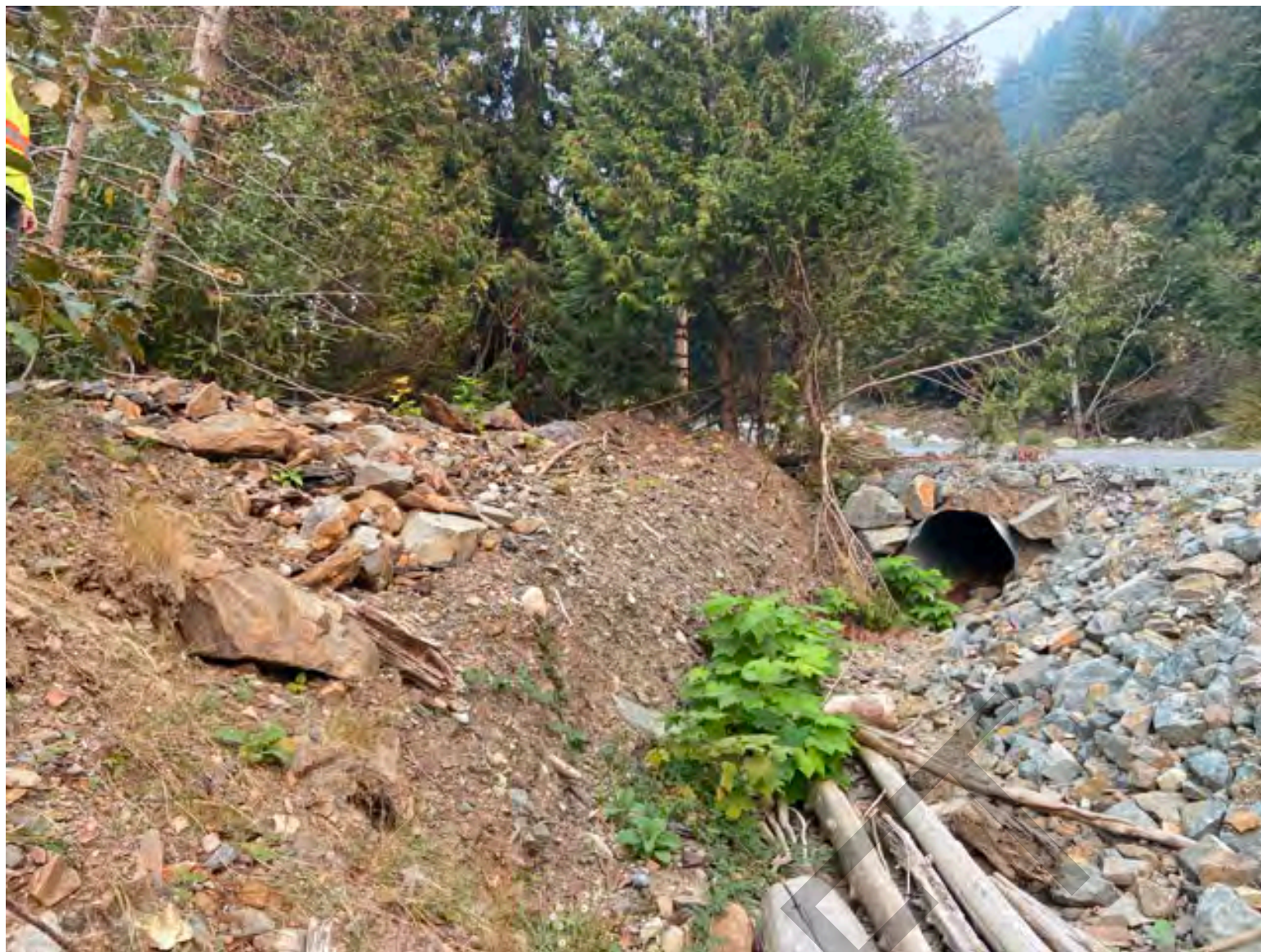
Photo 6 DF3-View east-northeast of terrain on the east side of Rockwell Drive and temporary works including ditching and riprap installation following the 2021 atmospheric river event
