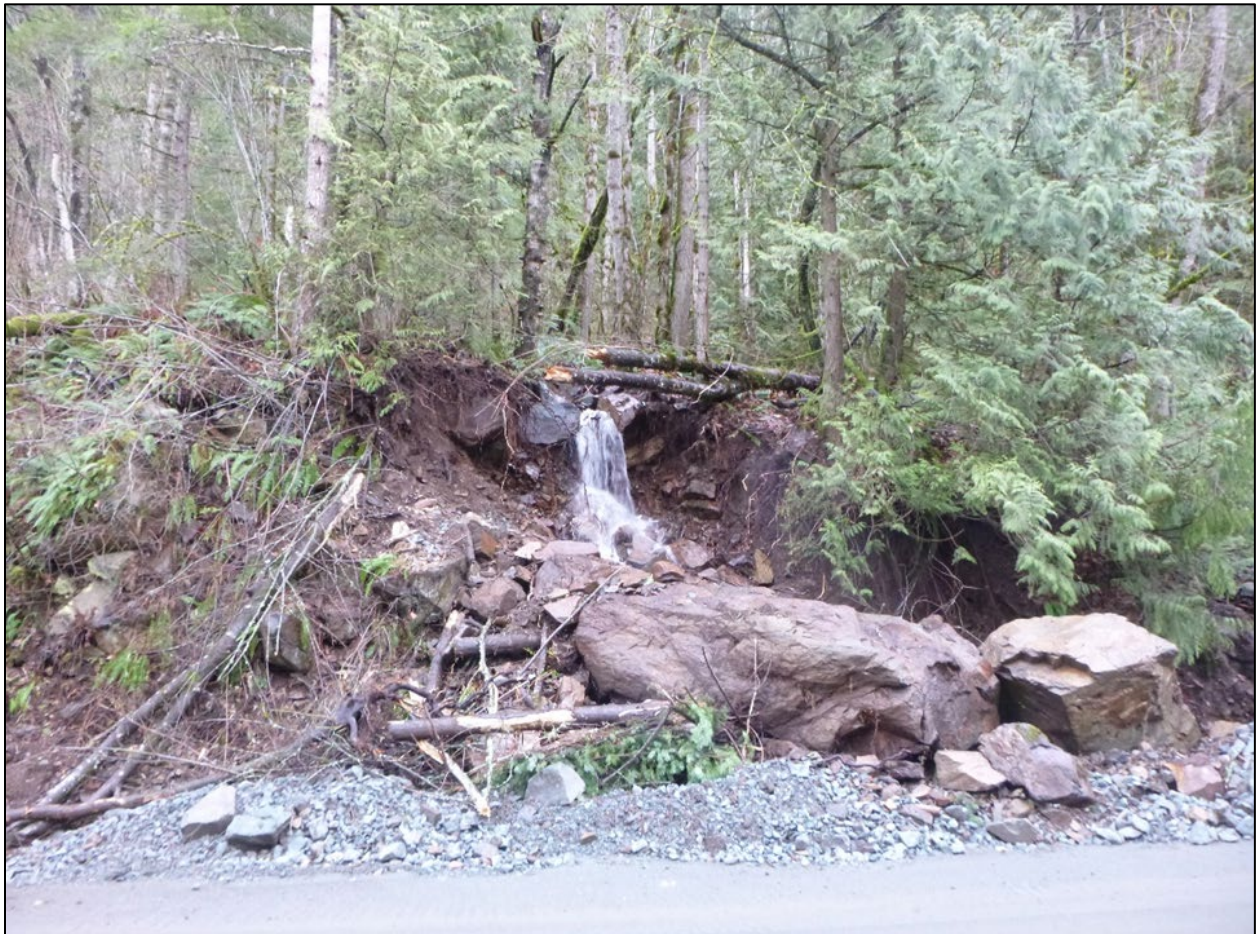
Figure 2 Watercourse avulsion at Site DF3 (December 14, 2021).
