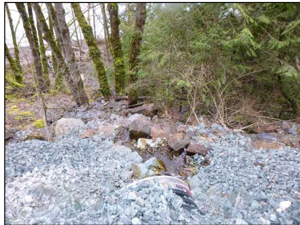
Photo 4: Rockwell Drive culvert outlet.
