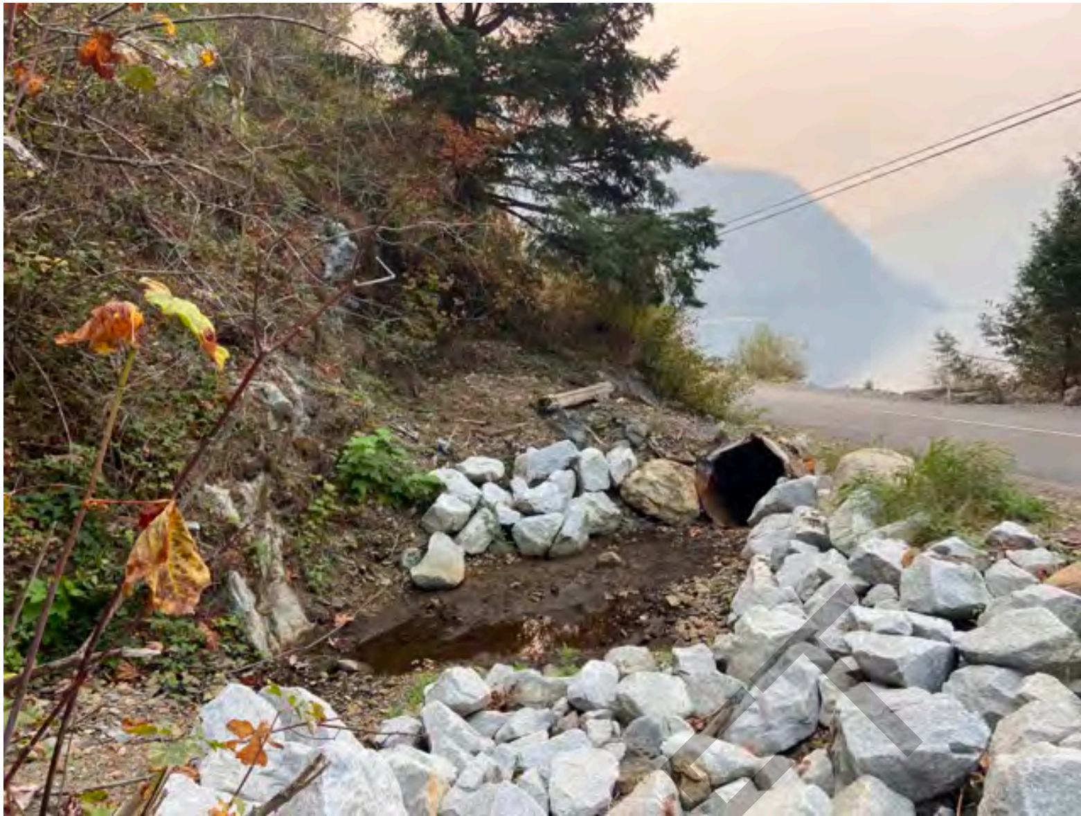
Photo 4 DF2 - View east-northeast of washout debris on an existing berm on the east side of Rockwell Drive.
