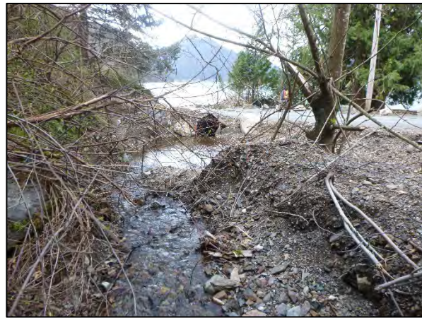
Photo 4: Downstream view of the Rockwell Drive culvert inlet where the roadside ditch and altered channel converge.
