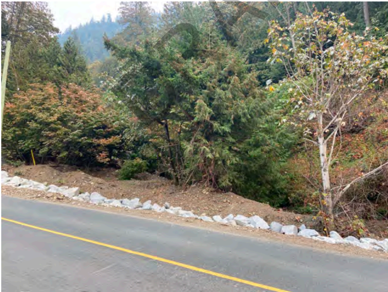
Photo 4 DF2 - View east-northeast of washout debris on an existing berm on the east side of Rockwell Drive.
