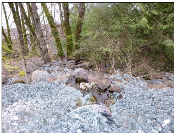
Rockwell Drive culvert outlet.
