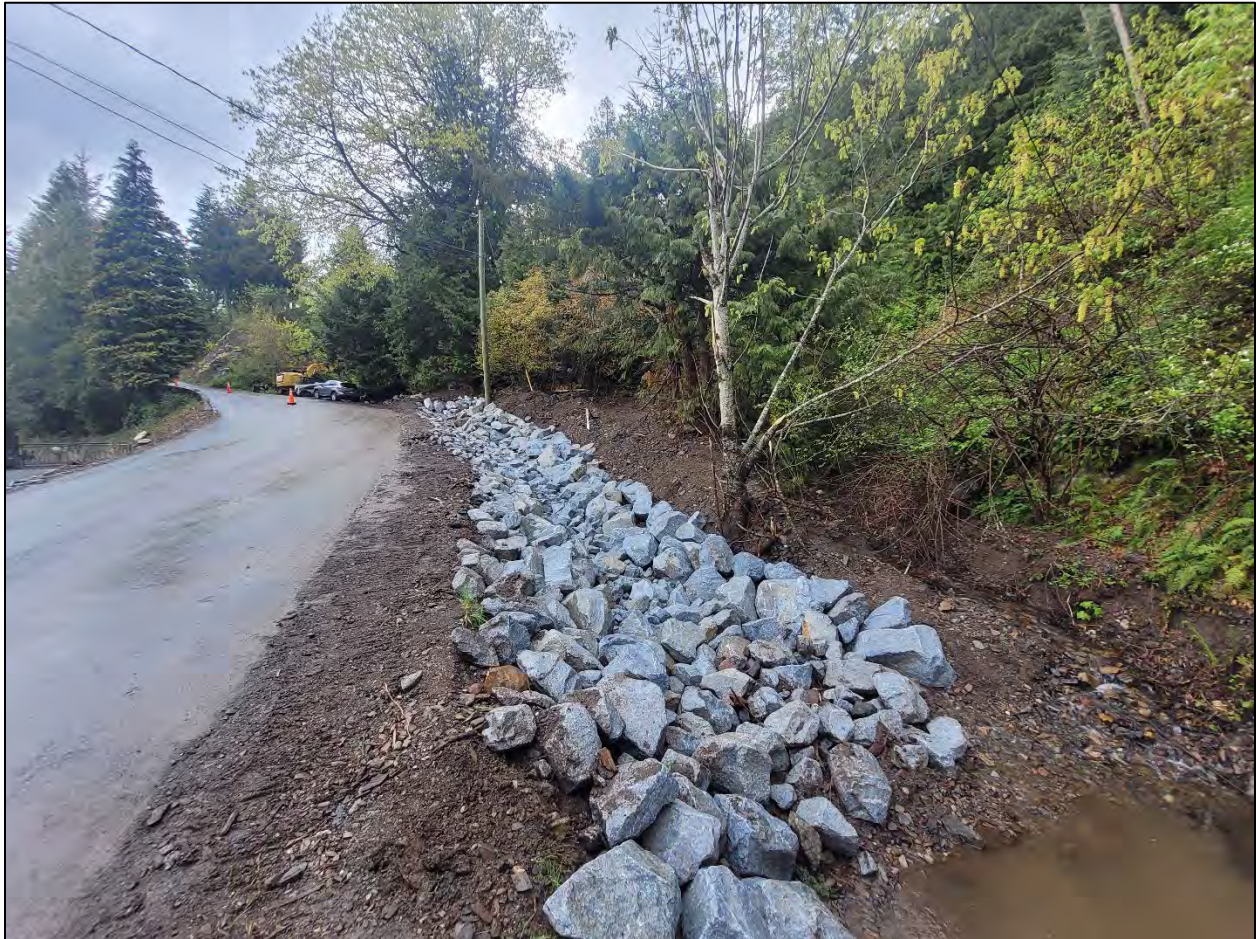
Figure 7 Short-term recovery works at site DF2 (April 26, 2022).
