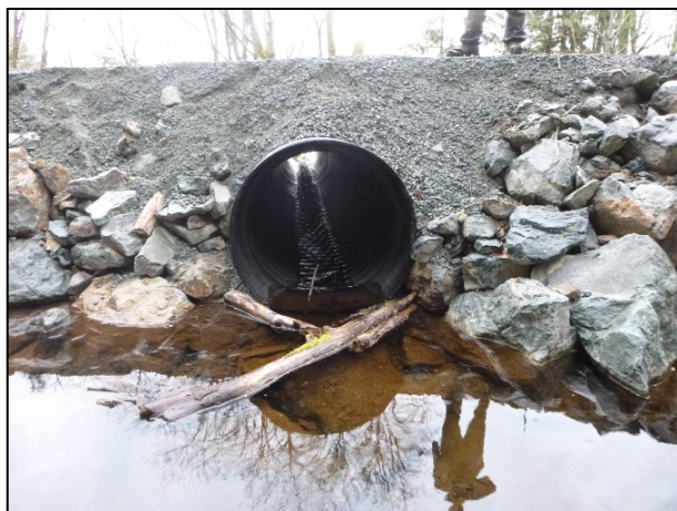
Rockwell Drive culvert inlet.
