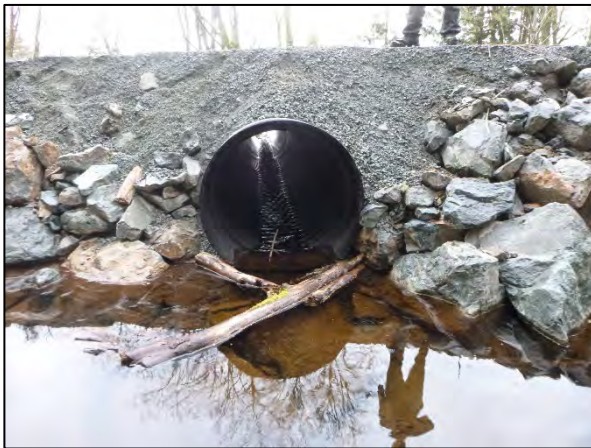
Photo 3: Rockwell Drive culvert inlet.
