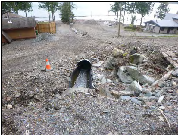
Photo 3: Downstream of Rockwell Drive the DF1 watercourse is culverted on private property.
