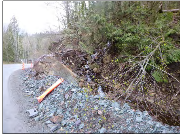
Photo 2: Creek avulsion directed back to the south via a berm along Rockwell Drive.
