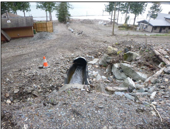
Downstream of Rockwell Drive, the DF1 watercourse is culverted on private property.
