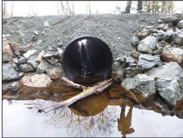
Rockwell Drive culvert inlet.
