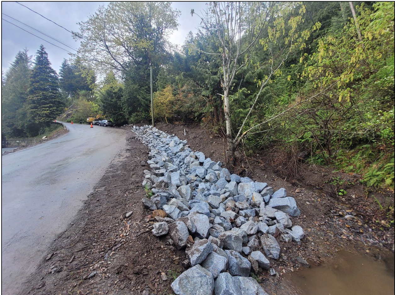
Figure 7 Short-term recovery works at site DF2 (April 26, 2022).
