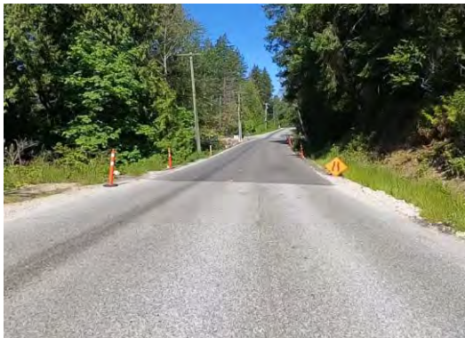
Figure 7: Redrooffs Rd – Looking west towards culvert crossing
