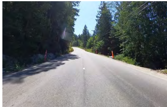
Figure 6: - Redrooffs Rd – Looking east from culvert crossing
