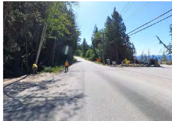
Figure 8: Redrooffs Rd – Looking east towards culvert crossing
