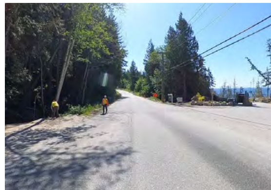
Figure 8: Redrooffs Rd – Looking east towards culvert crossing
