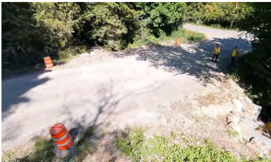
Figure 11: Beach Ave – Culvert crossing
