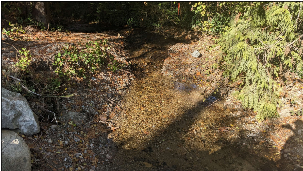
Photo 3. Channel conditions post-construction.
