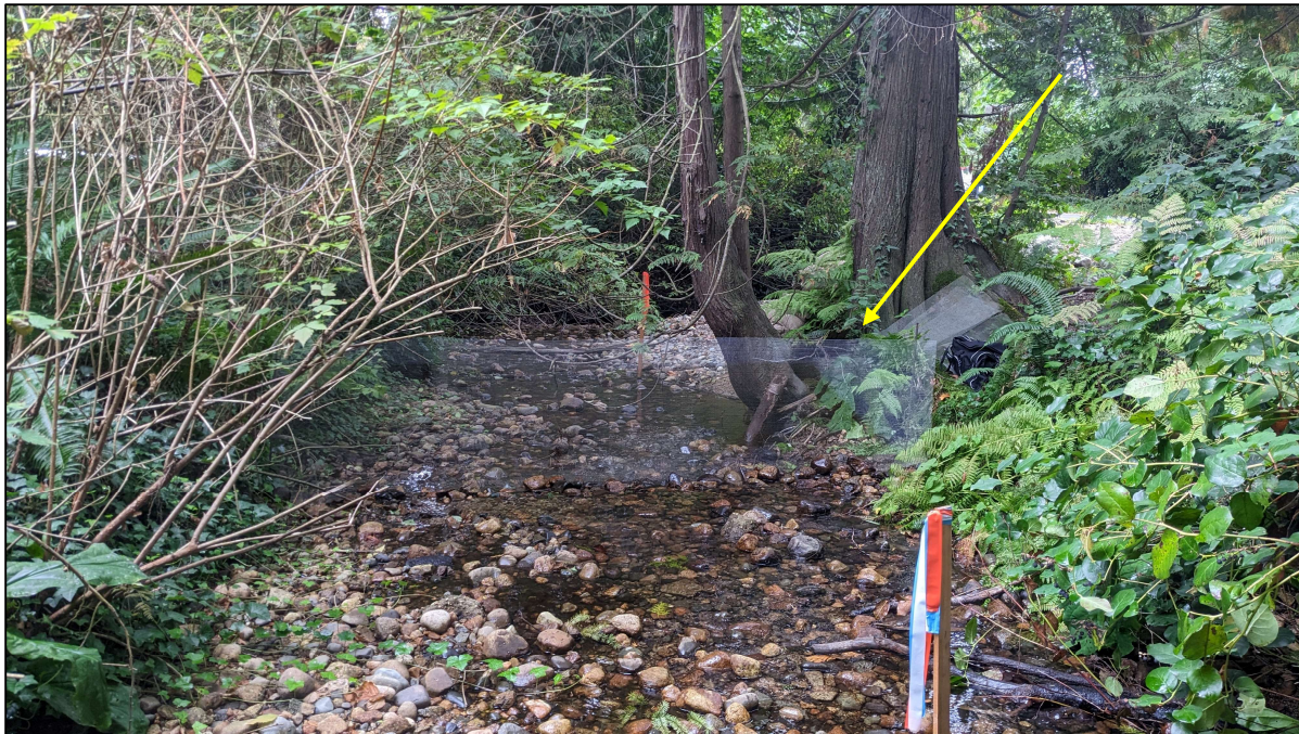
Photo 1. Viewing the work zone behind the fish barrier net.
