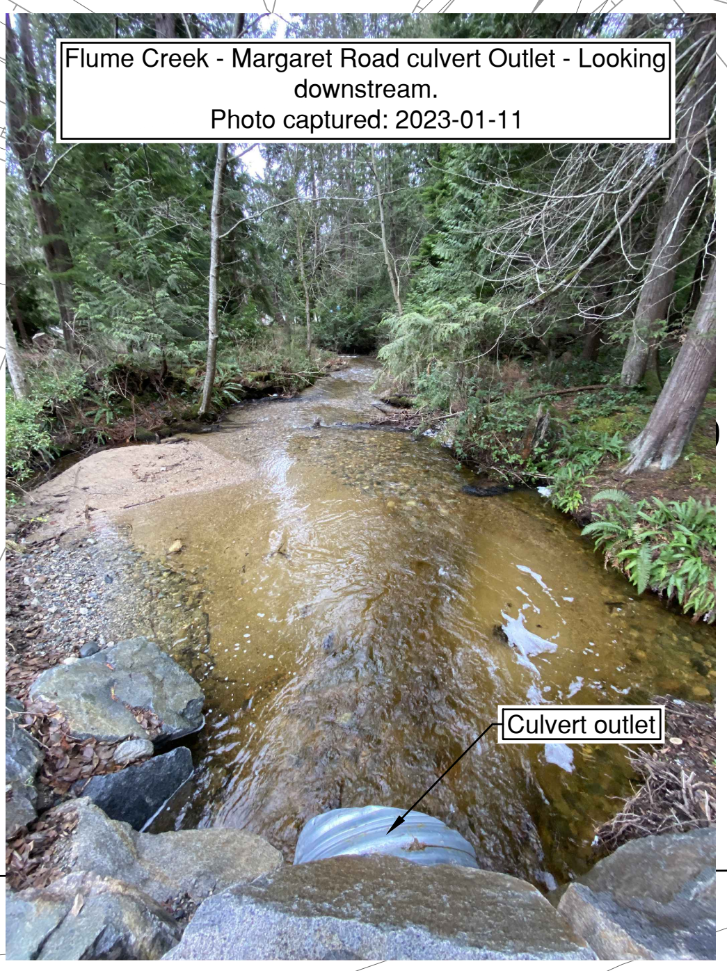
Flume Creek - Margaret Road culvert Outlet - Looking downstream. Photo captured: 2023-01-11
