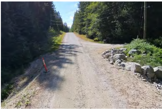
Figure 11: Day Rd at Clack Creek - Looking West
