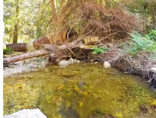
Figure 10: Day Rd – Clack Creek Downstream
