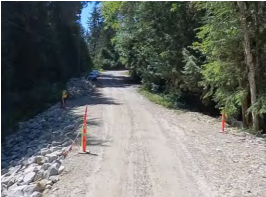
Figure 5: Day Rd at Gough Creek - Looking West
