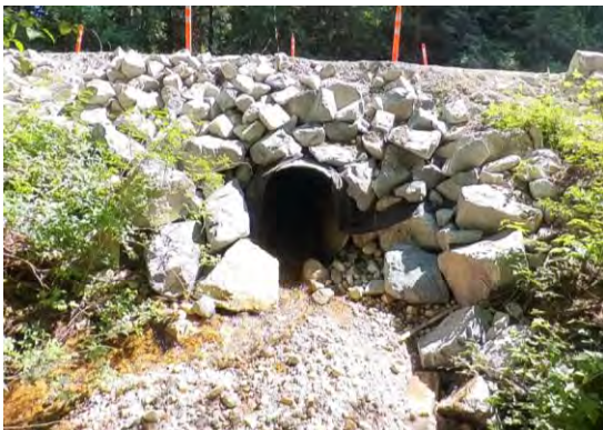
Figure 7: Day Rd – Clack Creek Inlet
