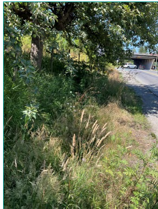
Photo 4. Looking north into the Project footprint at instream conditions of the unnamed ditch towards the King Road and Riverside Road intersection.
