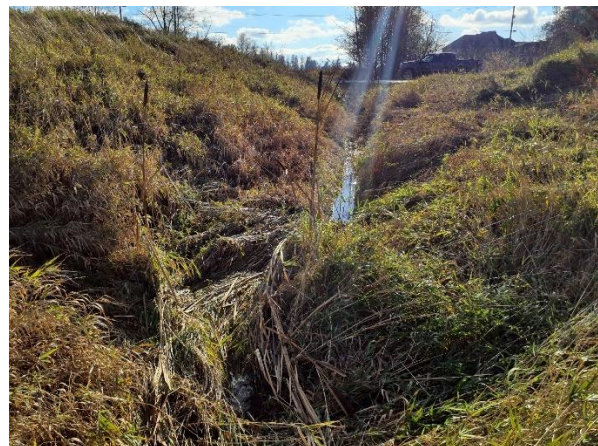
Photo 8. Class B watercourse located within the highway median.
