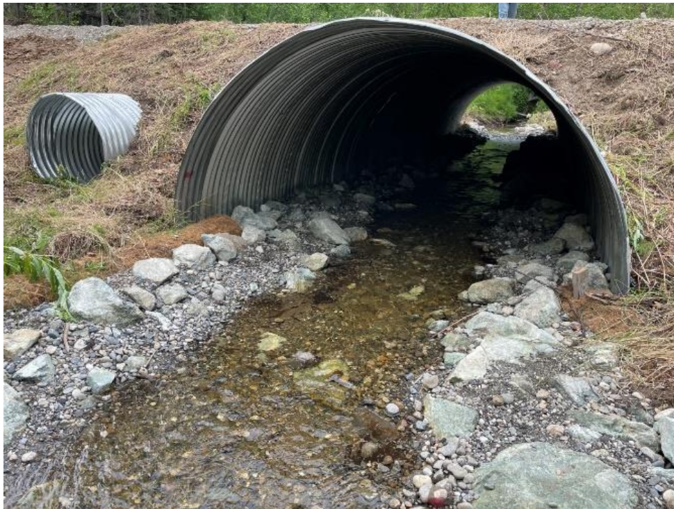
Figure 5. Example of embedded culvert.
