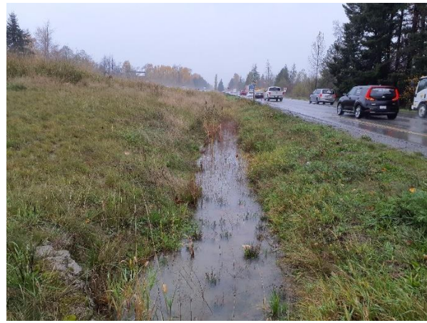
Photo 2. Class B ditch in the highway median.
