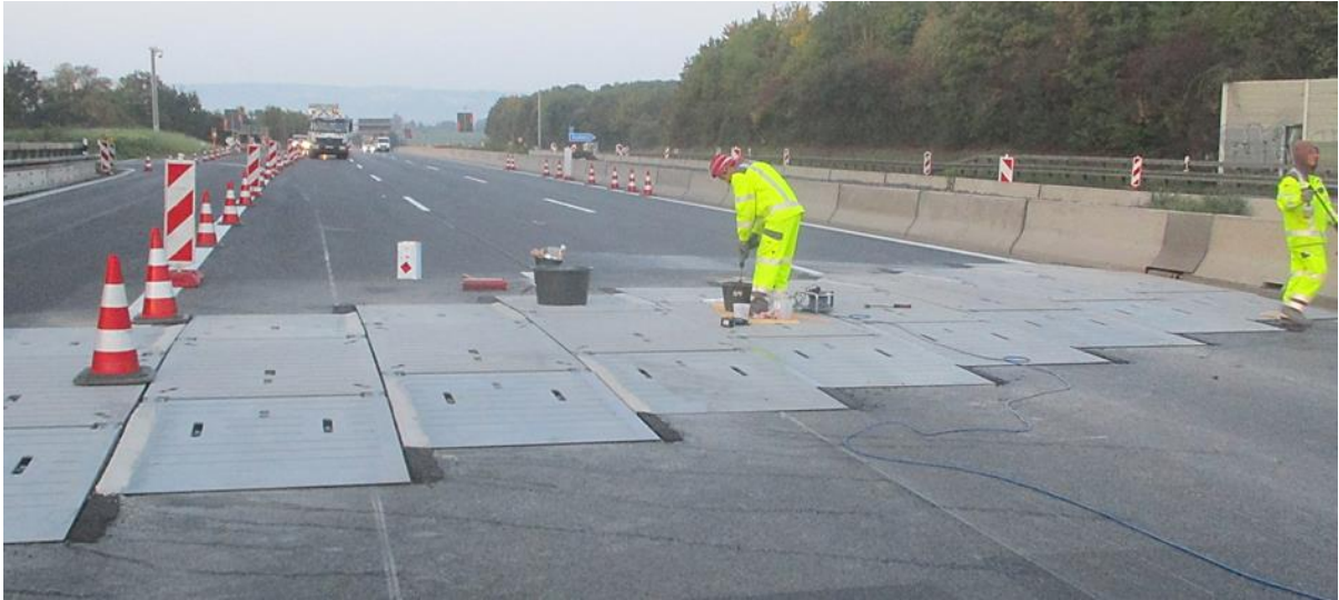
Figure 1: Illustration of MMBS System installation on construction site
