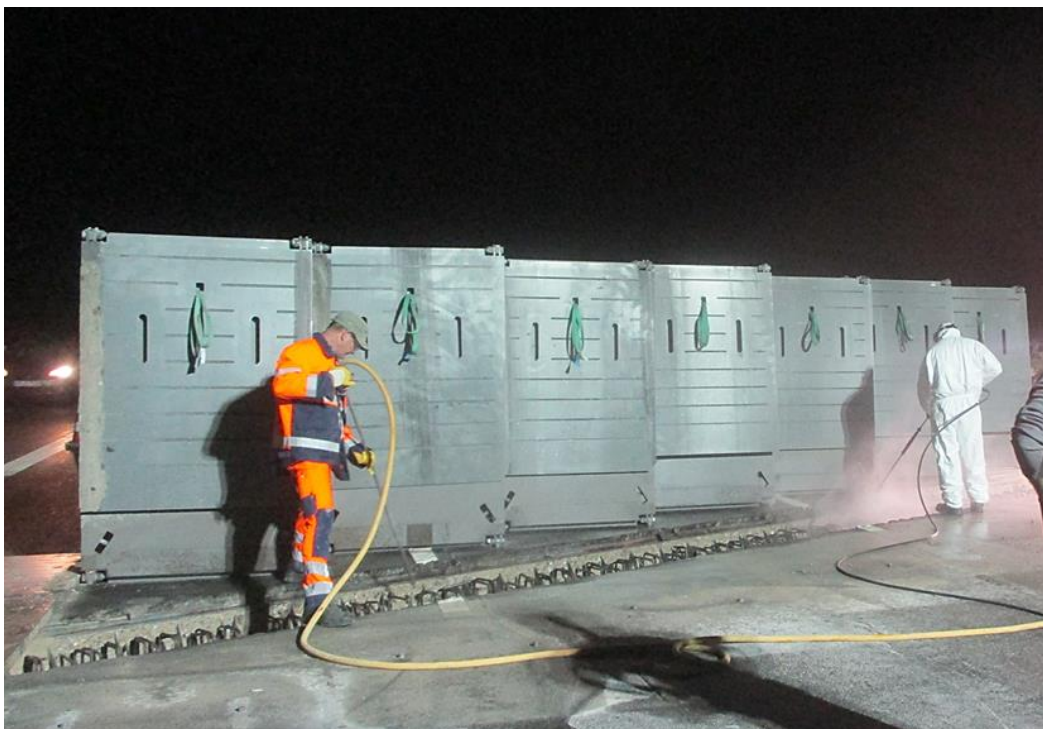
Figure 2: MMBS System lifted up
