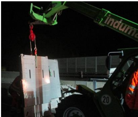
Figure 15: schematic figure opening and closing with steel rope and round slings
