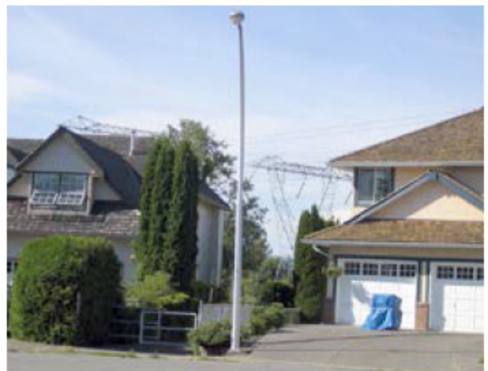
In this image, the visual impact of power lines is very strong, as little attention has been paid to varied orientation or the use of landscaping to 'hide' the towers. Photo: Google 2016.
