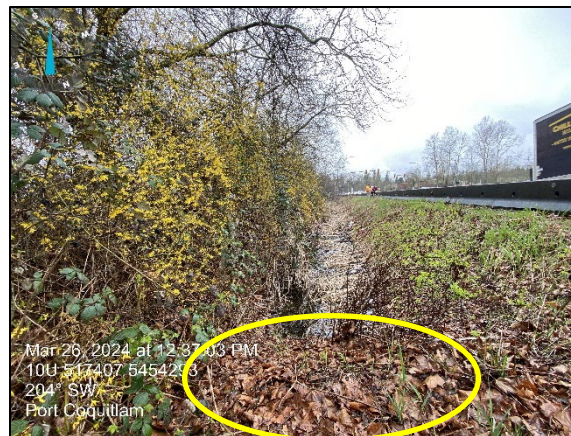
Photo 6.4 View of the ditch from on top of the berm (yellow circle) facing west towards the Broadway south intersection.
