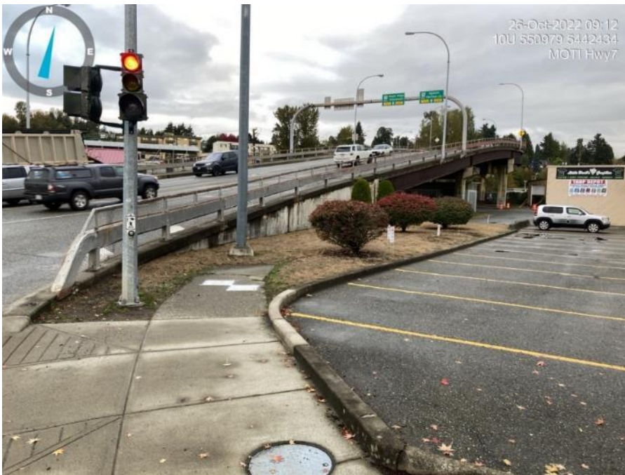
Photo 8: Glasgow Avenue Bridge connecting the northern and southern sites. Roadside vegetation consisting of grasses and ornamental shrubs.
