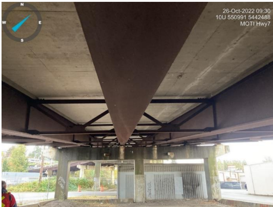
Photo 9: Potential bird and bat nesting/roosting habitat beneath the Glasgow Avenue Bridge.
