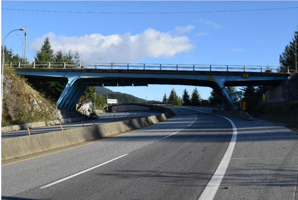
Exhibit 2.2-1: Eagleridge U/P Looking East
