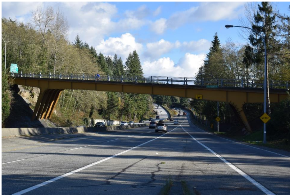
Exhibit 2.4-1: Westmount U/P Looking East
