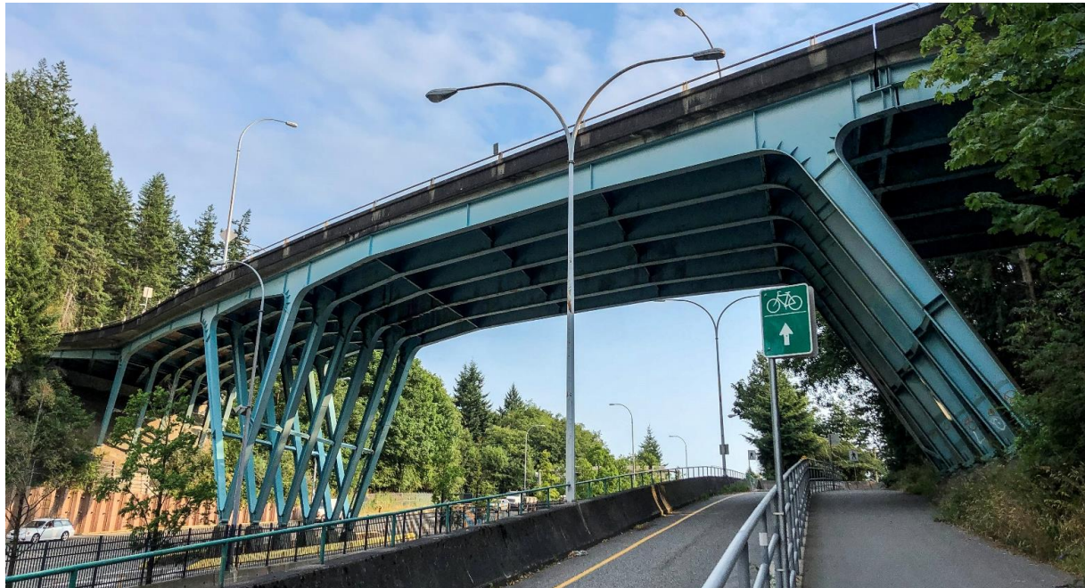
Exhibit 2.1-1: Horseshoe Bay U/P Looking South
