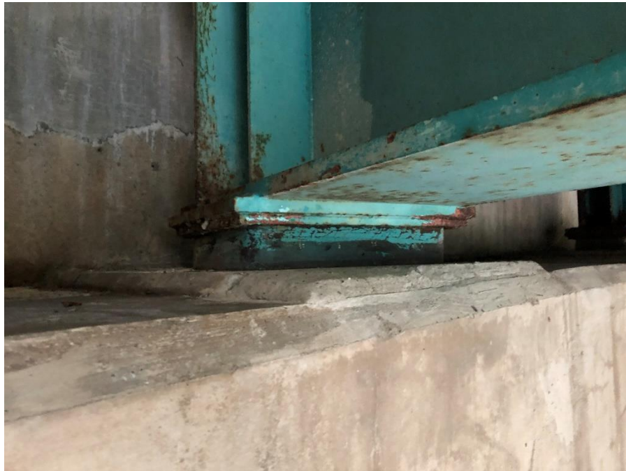
Exhibit 3.1-8: Abutment Bearing W6, Typical West Abutment Bearing Condition.
