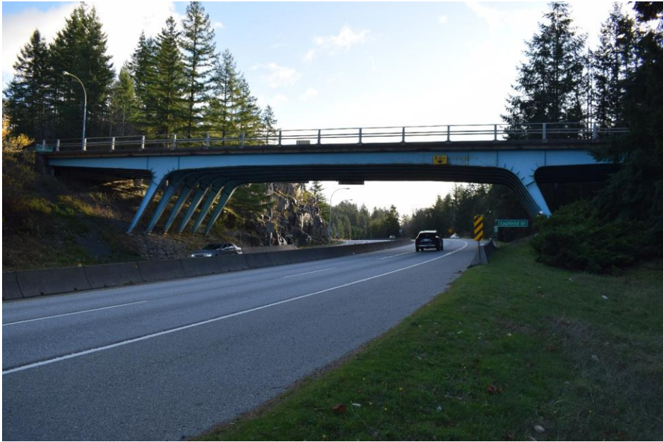
Exhibit 2.3-1: Caulfield U/P Looking East
