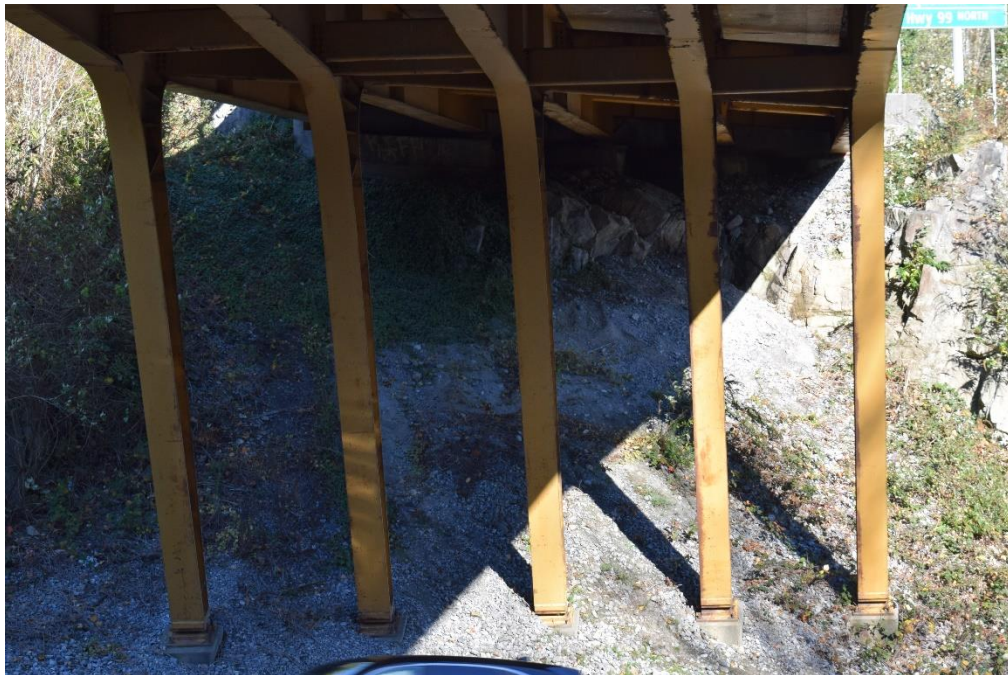
Exhibit 3.4-10: North Abutment Pier Legs, Fair to Good Condition
