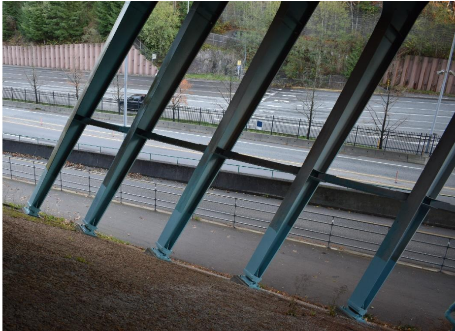
Exhibit 3.1-13: West Inclined Pier Legs Observed in Good Condition
