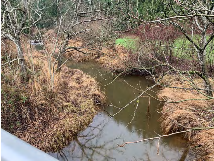
Photo 3 View upstream of Miami Creek from the highway bridge crossing.
