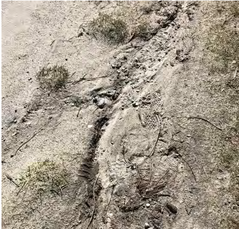
Photo 9 Evidence of north to south drainage along the west side of Sechelt Inlet Road. Photo taken facing south near the intersection with Tsulich Drive at 104+60.
