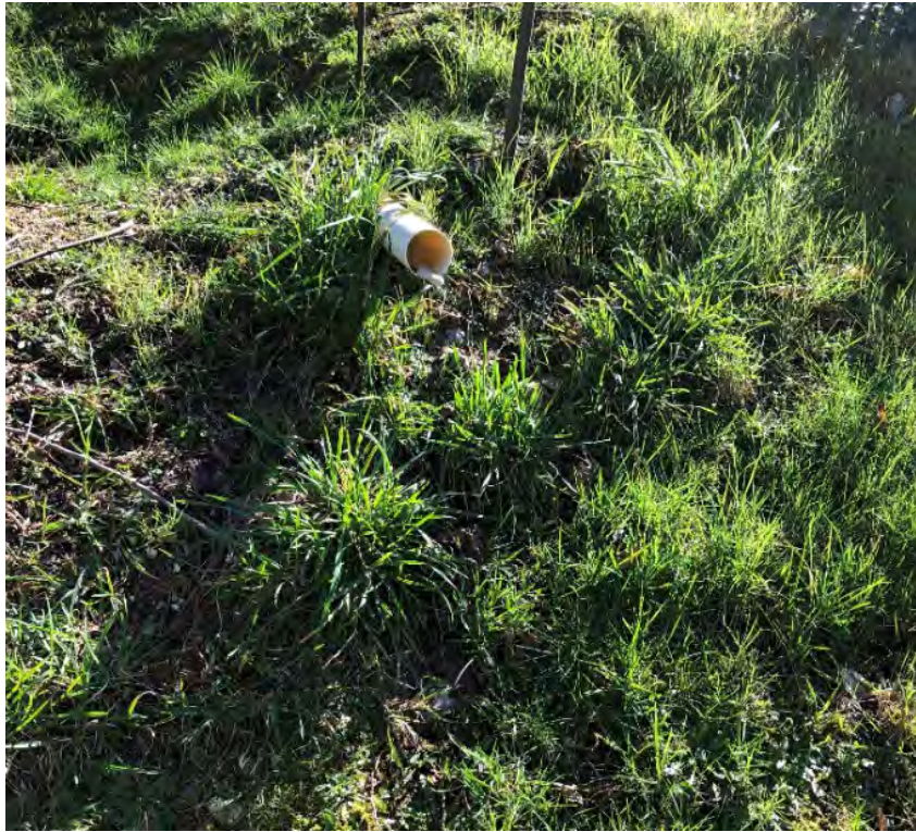
Photo 11 A drainage pipe observed conveying water from a residential property on the eastern side of Sechelt Inlet Road. Photo taken at 100+90 near Sechelt Inlet Road and Xenichen Avenue, facing east.
