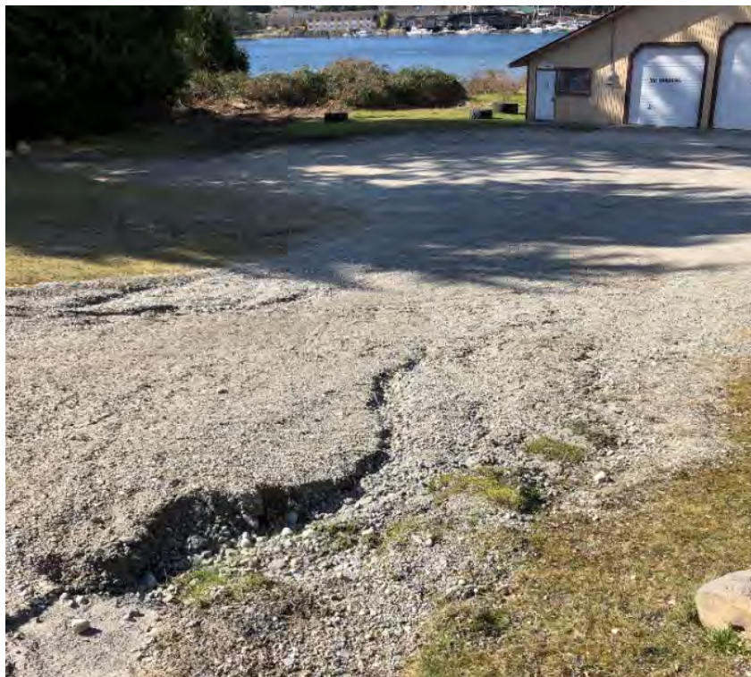
Photo 10 Surface drainage from Sechelt Inlet Road westwards down a gravel driveway approximately 3 meters south of the intersection with Tsulich Drive.
