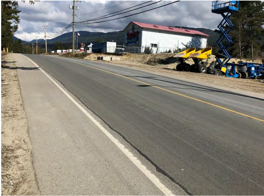
Photo 1 Sechelt Inlet Road, facing northeast.
