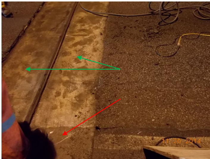
Description: Joint 14 Post Demolition
