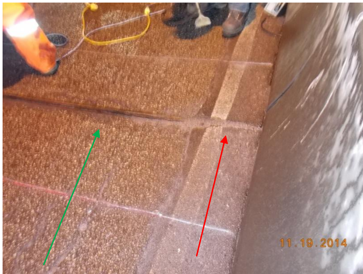
Description: Joint 12 Prior to Demolition
