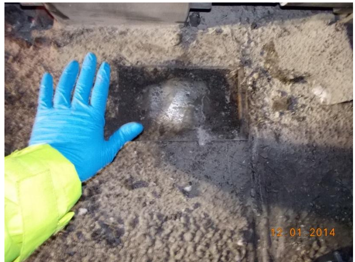
Description: Joint 8 During Primer Sampling
